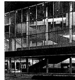
// HEMLOCK-CLAD FEATURE STAIR BEHIND CURTAIN WALL
