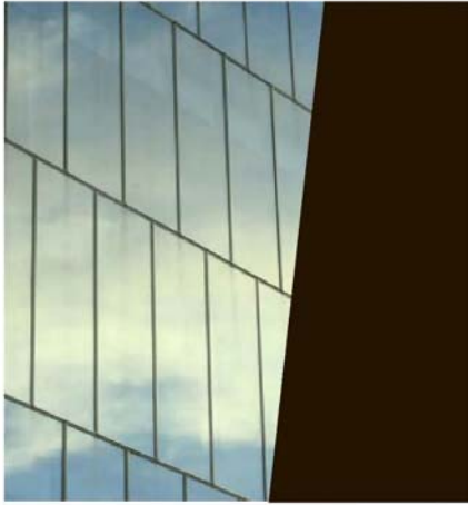
▲ // DOUBLE-GLAZED CURTAIN WALL AND WINDOWS STRUCTURAL SILICONE / DARK BRONZE MULLIONS
