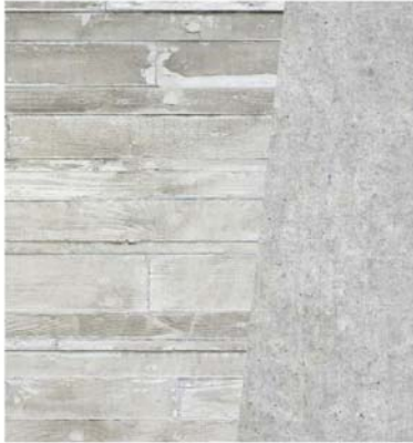
▲ // CAST-IN-PLACE CONCRETE BOARD-FORMED / SACK FINISH
