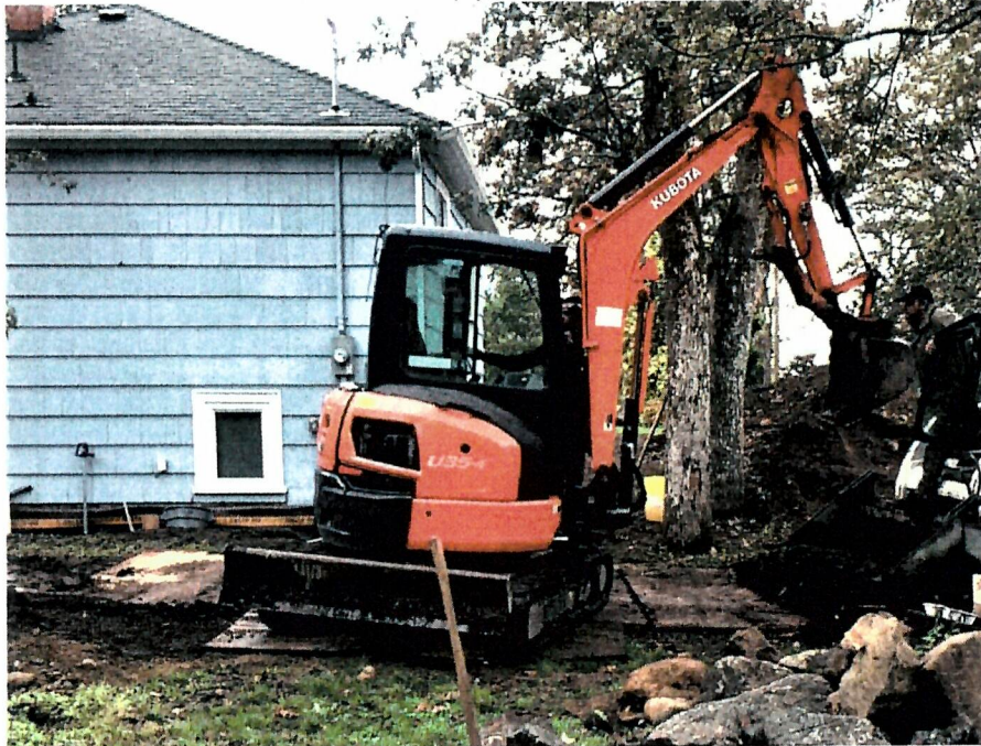
Image 14: Rubber tracked mini excavator on plywood sheets.
