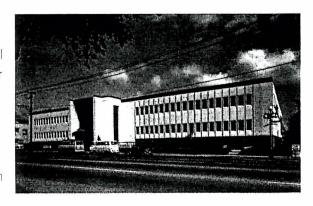
paper company and other tenants. The building is clad with precast concrete panels with built-in windows. The structural system consists of concrete slabs with capitals and drop panels, supported by concrete columns on a 24' grid. The original Victoria Press building and its façade will be preserved for its historic character.
