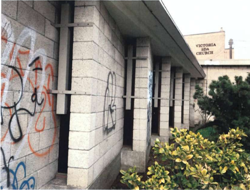
Saw-tooth splayed concrete walls
