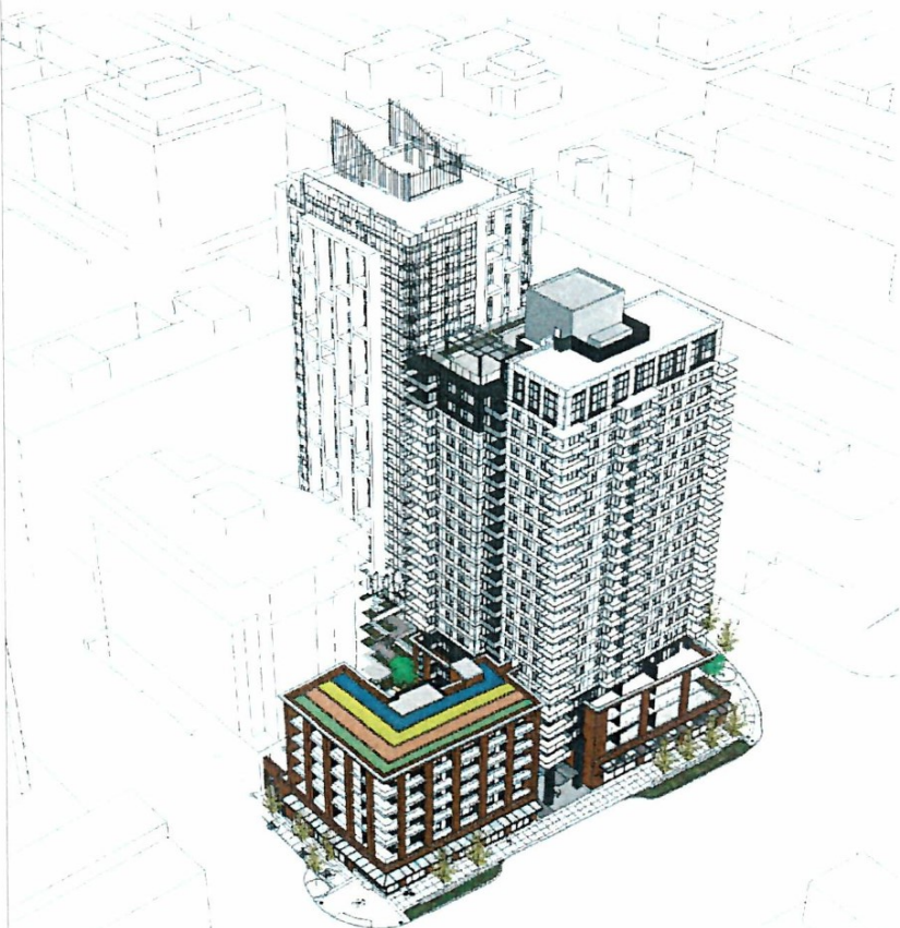
AERIAL VIEW LOOKING NORTH WEST
