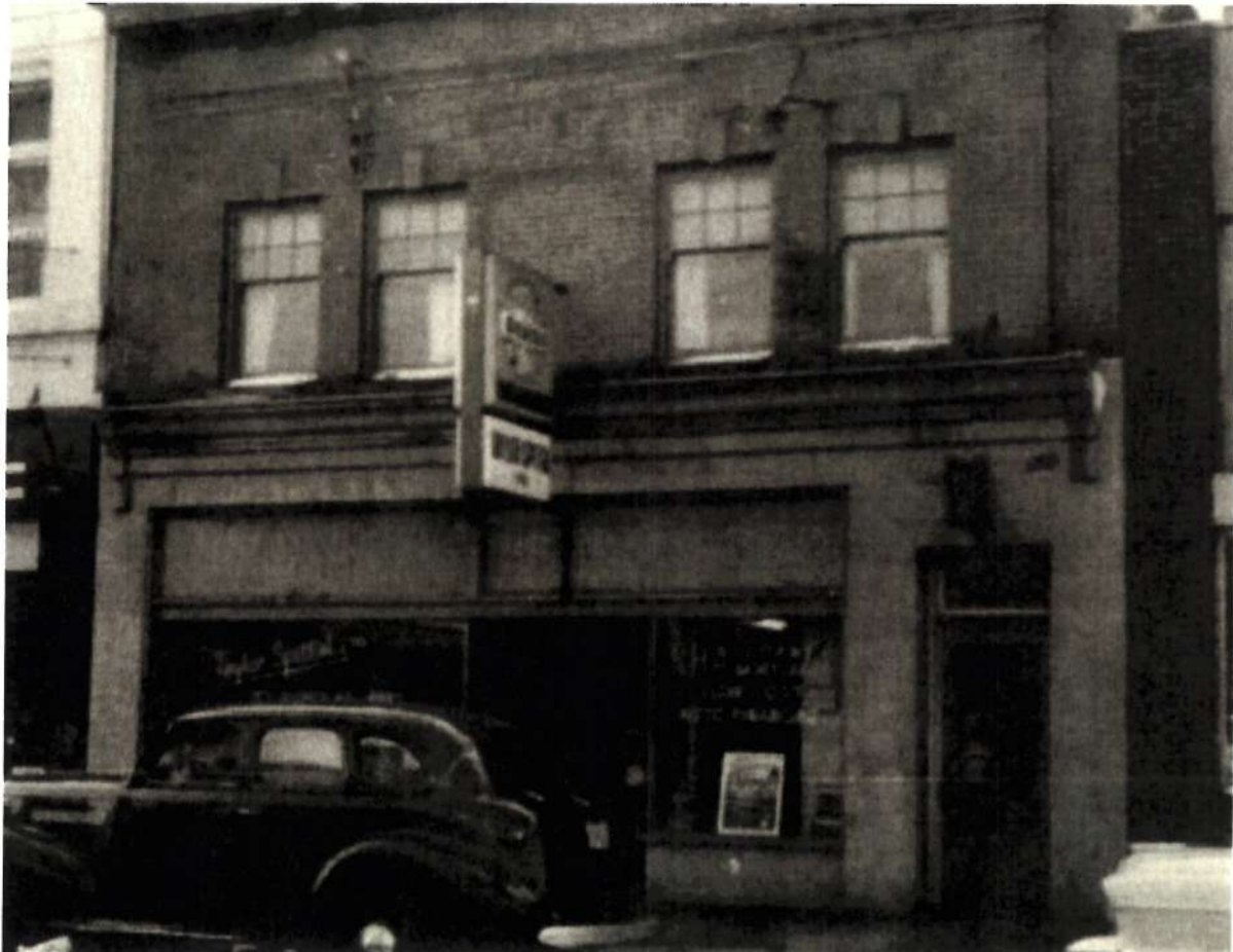
Detail photo showing original storefront at ground level, and double-hung wood windows at upper level. (City of Victoria Archives M03921_141)
