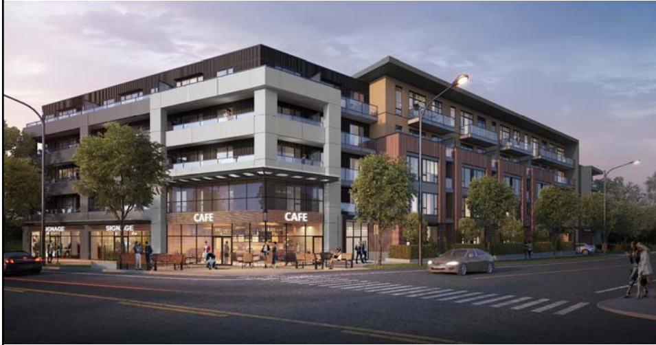
View from the corner of Gorge Road East and Irma Street
