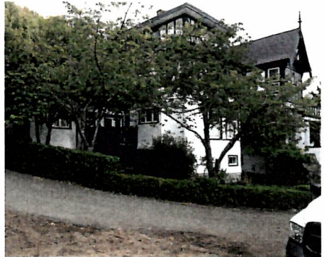
6 VIEW FROM SOUTH-WEST A-1 Star site screened by trees
