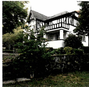
7 VIEW FROM SOUTH-EAST A-1 Principal entrance approach - new star not visible
