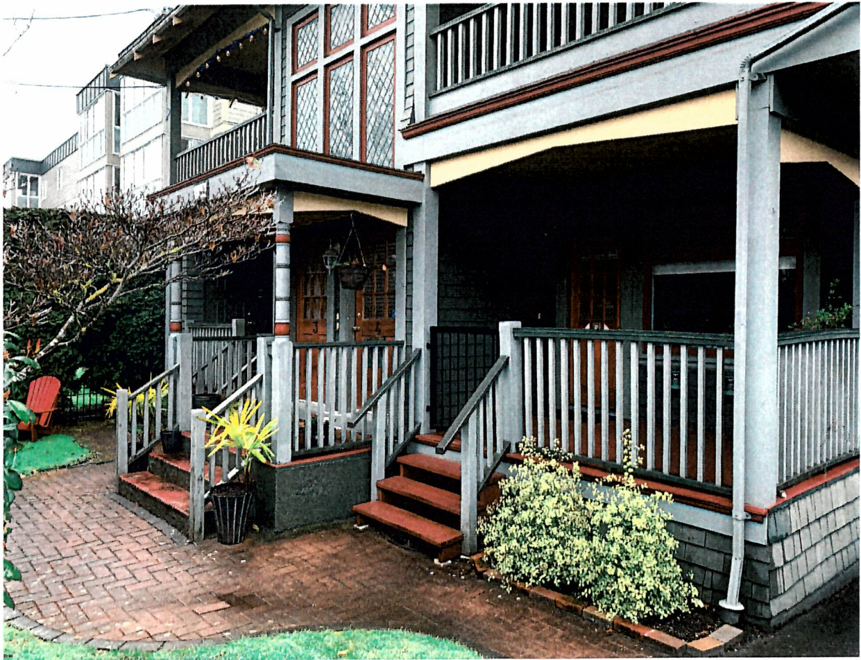
Front Elevation Closeup
