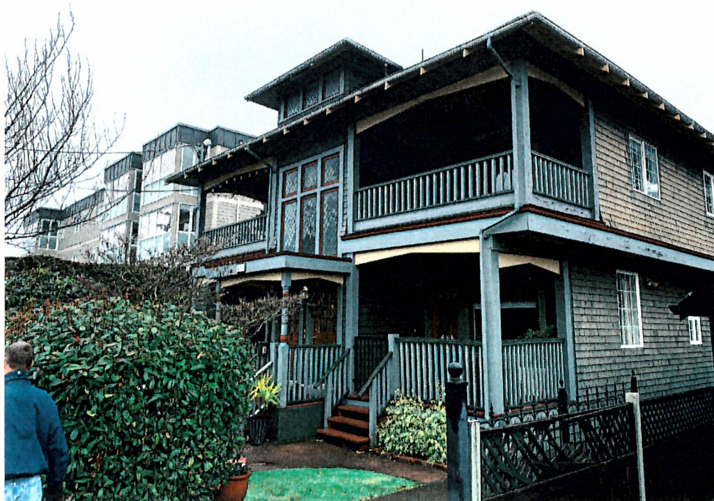
Angled view of Front Elevation with cantilevered second storey visible
