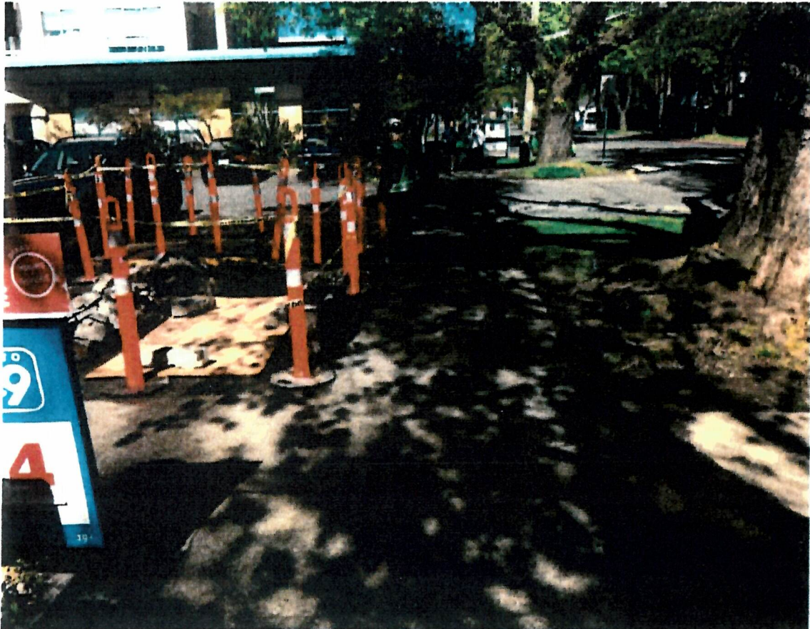
Pic. 1 – Location of exploratory excavation.
