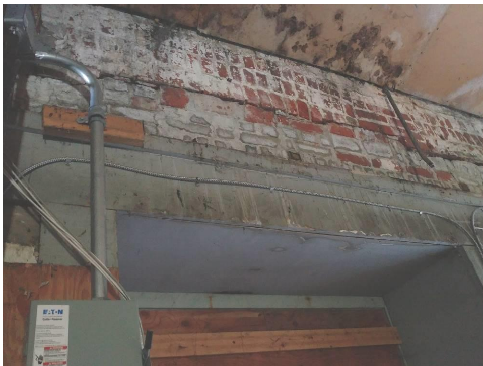
Segmental arch above altered front opening
