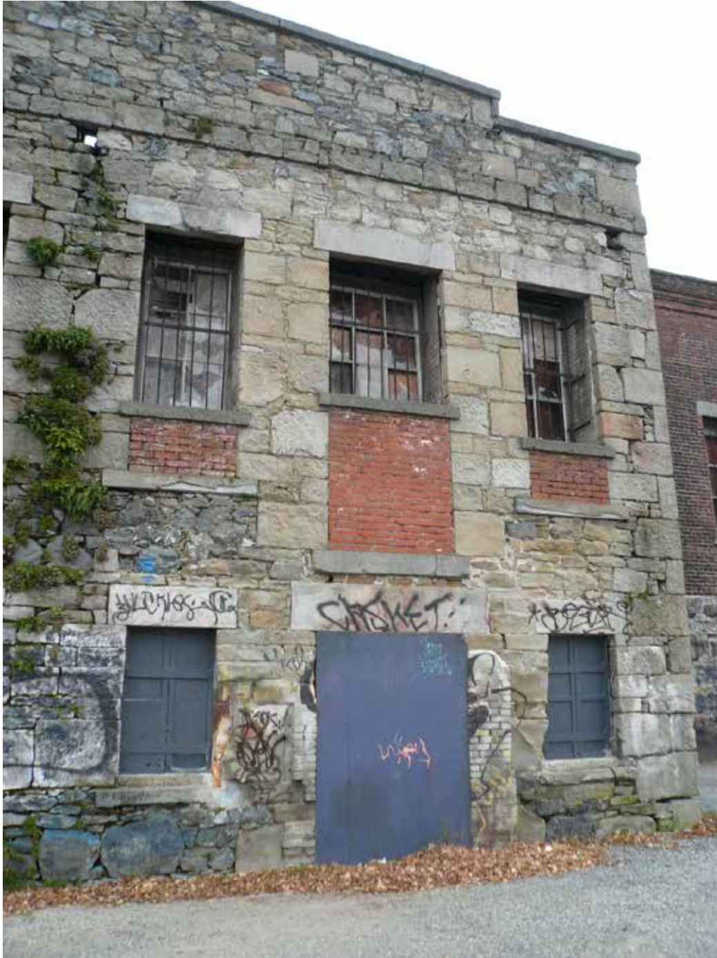
Rear elevation of the Fraser Warehouse showing openings altered using brick, changes to window assemblies, and general condition of masonry.
