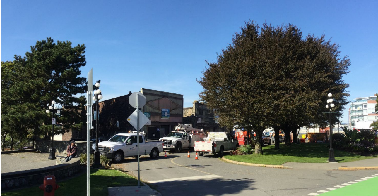
Photo 1. The subject site viewed from Wharf Street.
