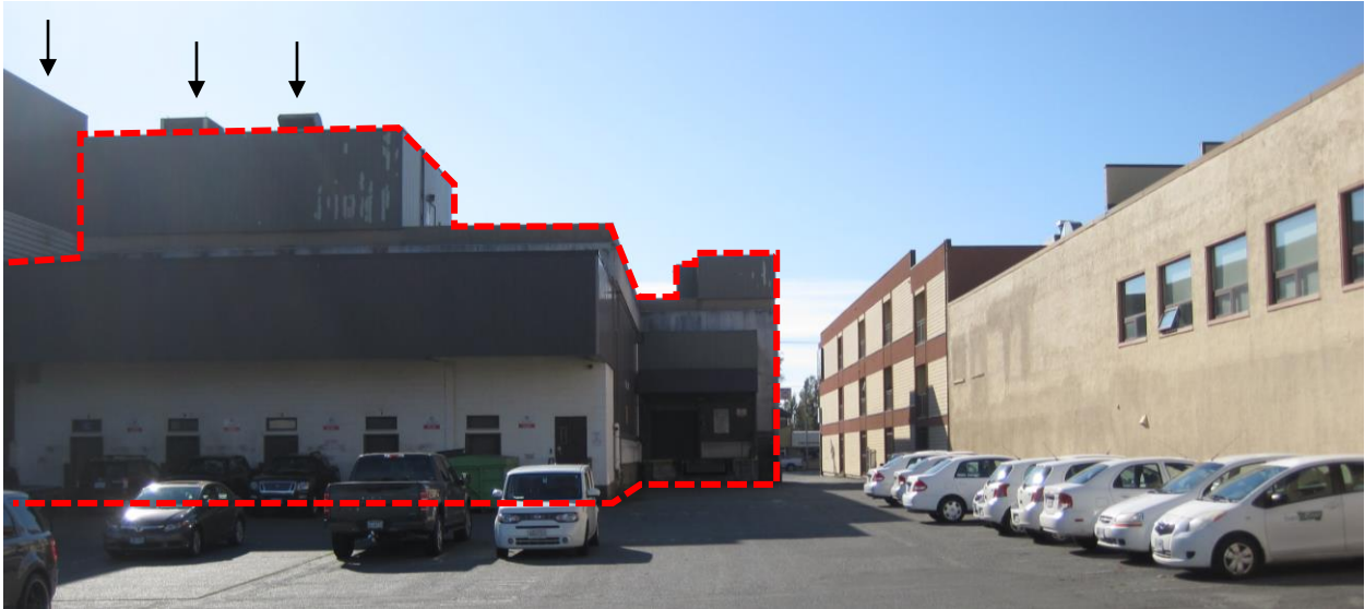
Rear (East) Elevation and Side (North) Elevation
