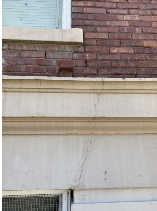
Crack in Brickwork
