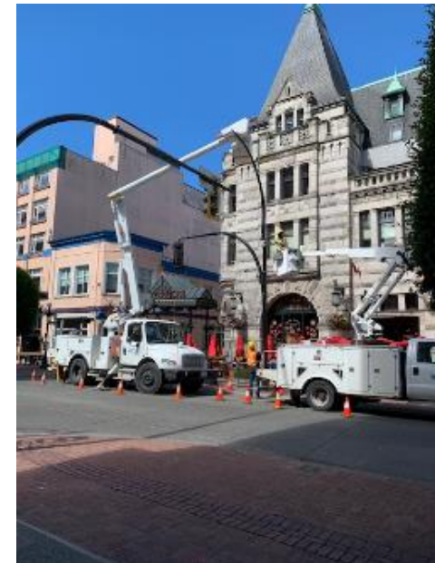
Traffic Signal Removal on Government Street at View Street as part of Build Back Victoria pedestrian priority initiative
