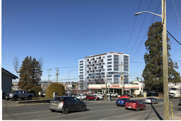
2 A0.4 View North-east across Burnside at Sulfand Road
