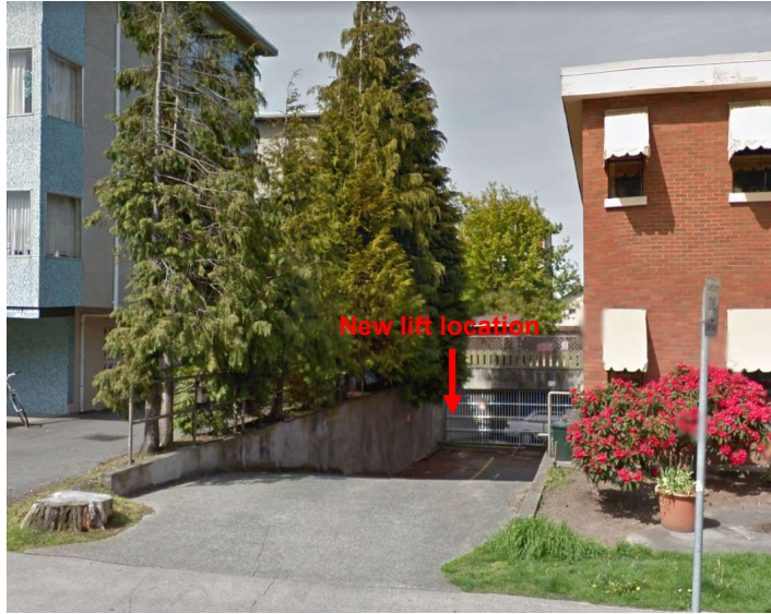
View of parking ramp
