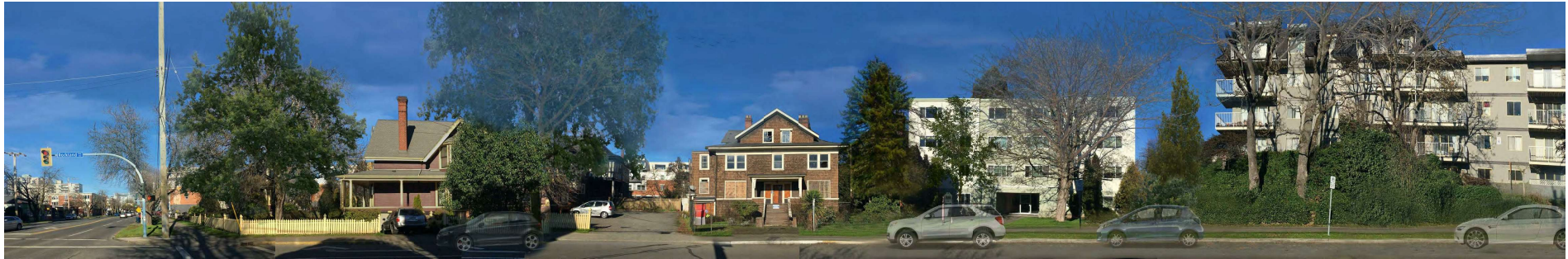
① STREET VIEW - EXISTING
