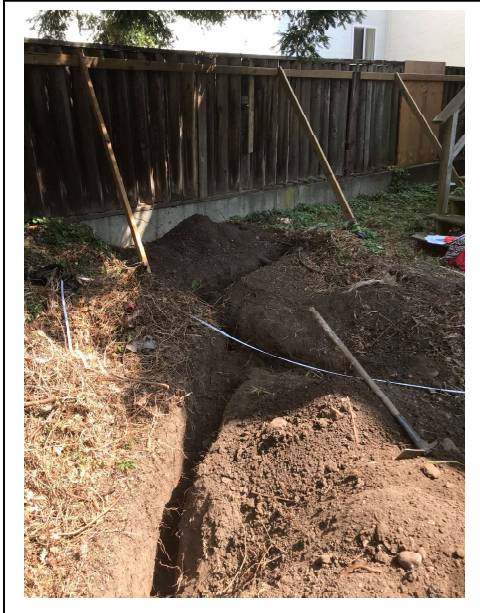
Excavation viewed from north west
