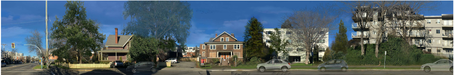
① STREET VIEW - EXISTING
