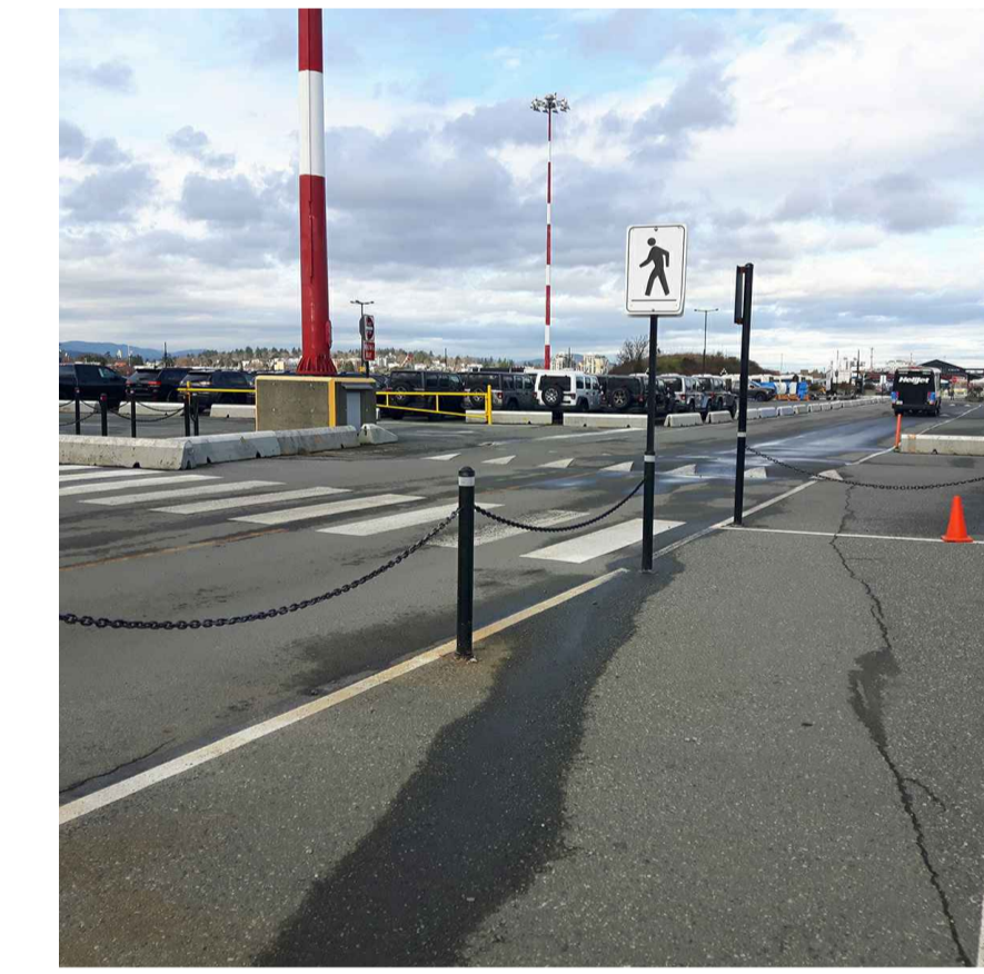
View from ramp landing to Crosswalk
