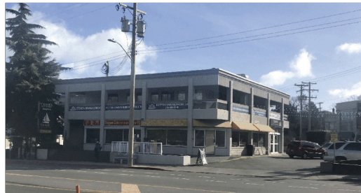
EXISTING BUILDING - FORT STREET
