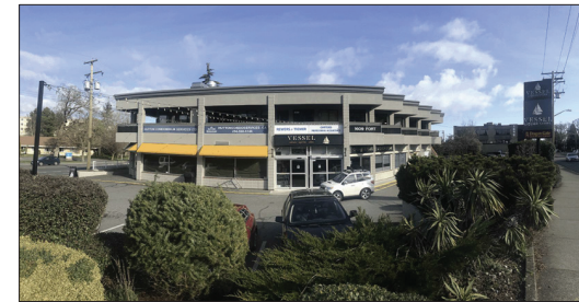
EXISTING BUILDING - OAK BAY AVENUE
