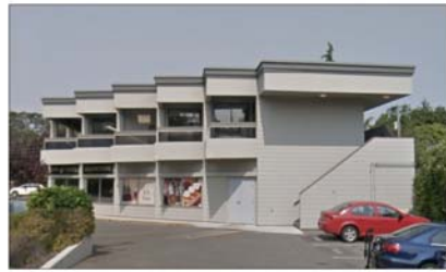
EXISTING VIEW FROM OAK BAY AVE
