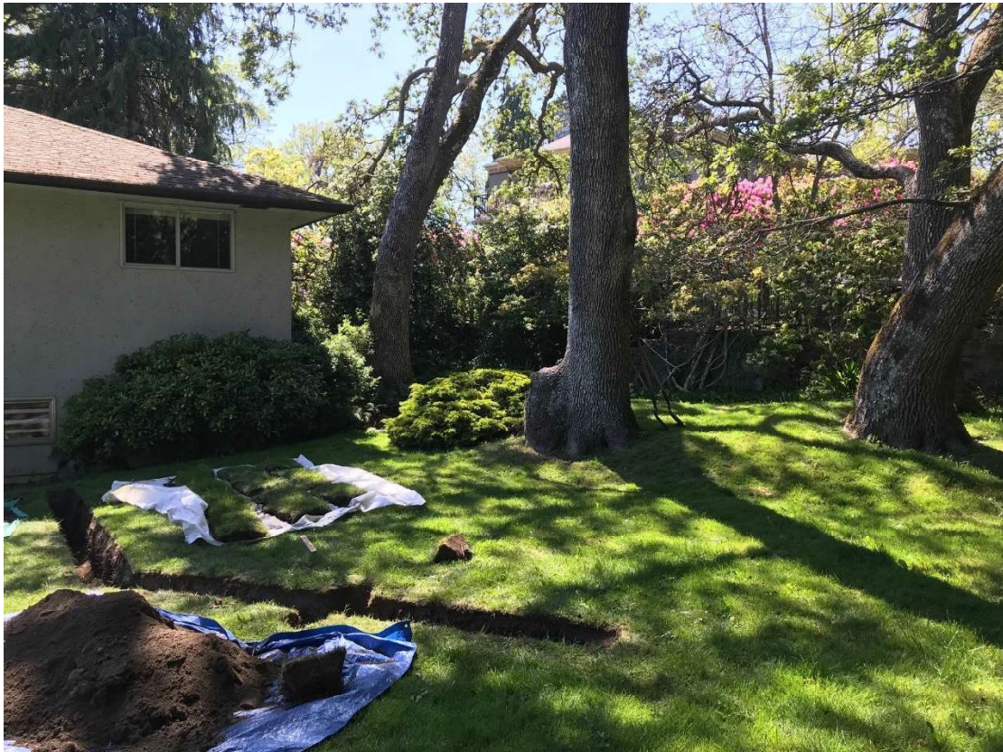
A trench was hand-dug at the approximate location of the proposed foundation excavation, 4.5m from Oak #201.
