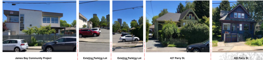
James Bay Community Project
