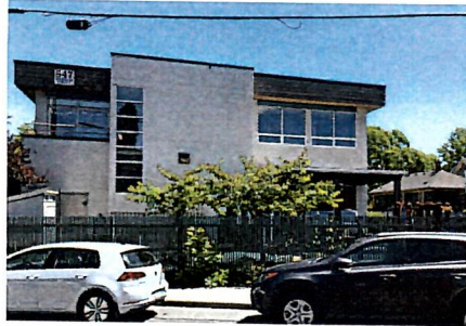
James Bay Community Project
