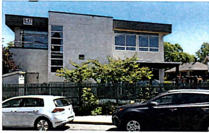
James Bay Community Project
