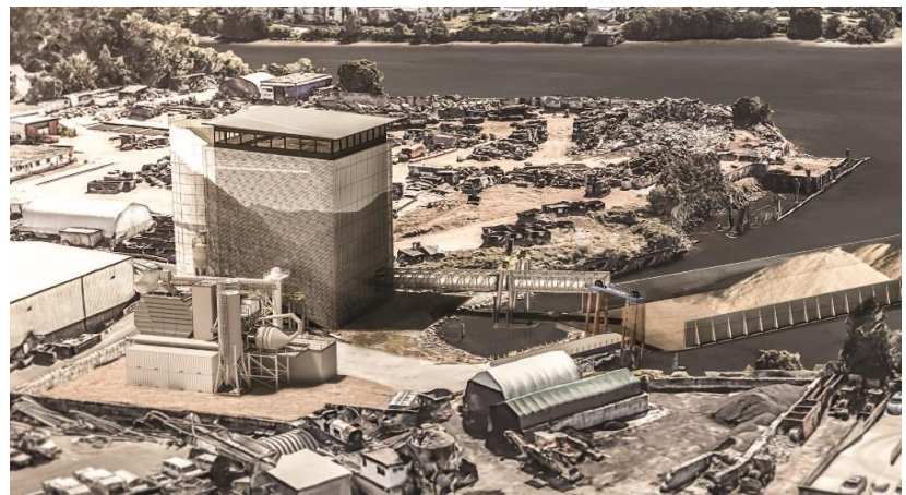
The new Trio site showing shipments arriving via barge. The large silo on the left will store aggregate and sand.
