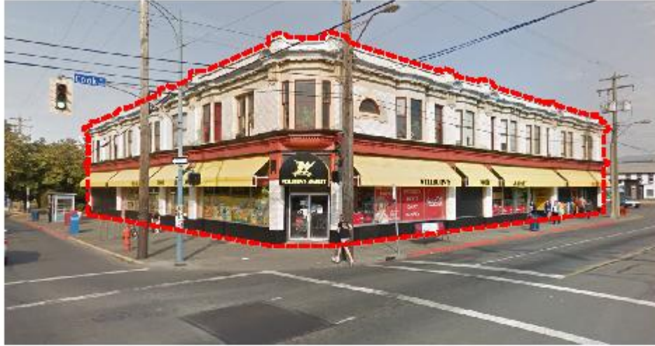
South and West Elevations Extent of building subject to designation outlined in red Note: Designation excludes awnings and canopies
