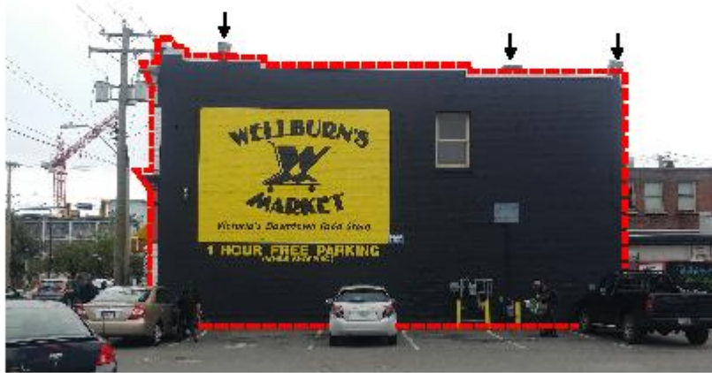
North (side) elevation Extent of building subject to designation outlined in red Note: Designation excludes rooftop lighting and mechanical equipment indicated by the arrows
