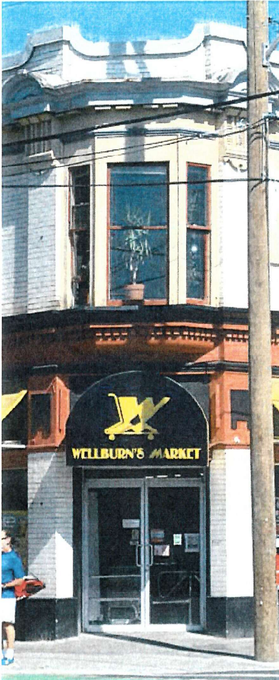
Above: Chamfered entry on ground floor with double doors and transom. Historic assembly has been replaced with aluminum assembly, including transom.
