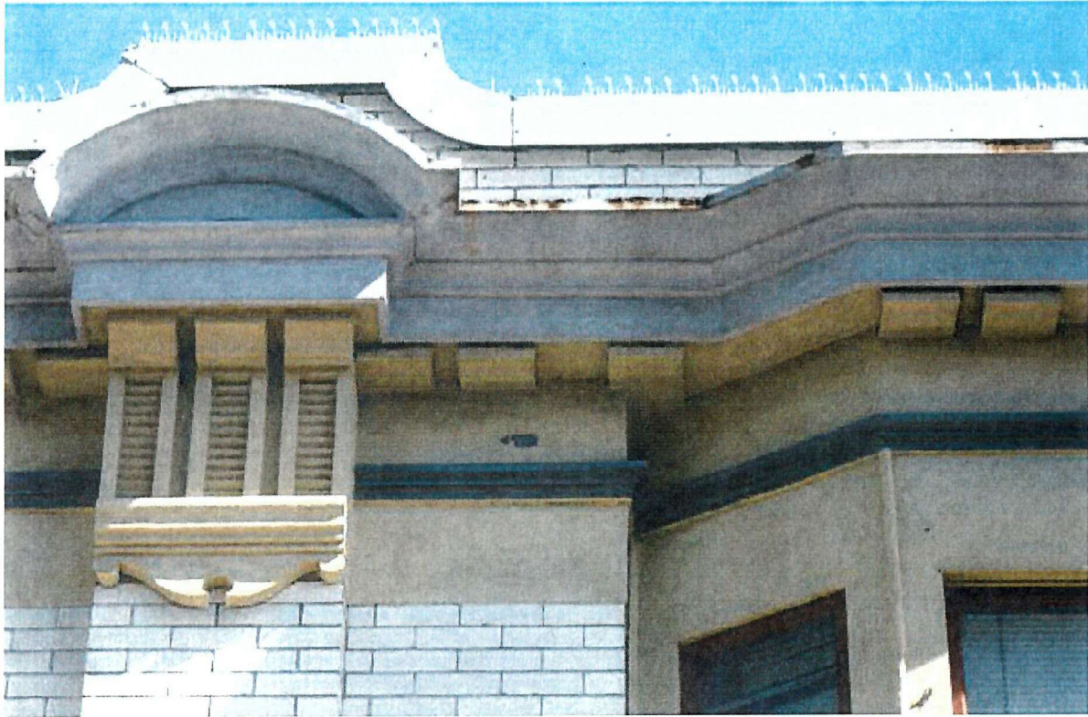
Above: Metal work of oriole windows, roof level cornice, top of brick pilasters, and parapet cap flashing. Paint failure evident and corrosion of drip edge on cap of cornice evident. Gap between parapet cap flashing and wall face noted. Bird spikes on parapet later addition.
