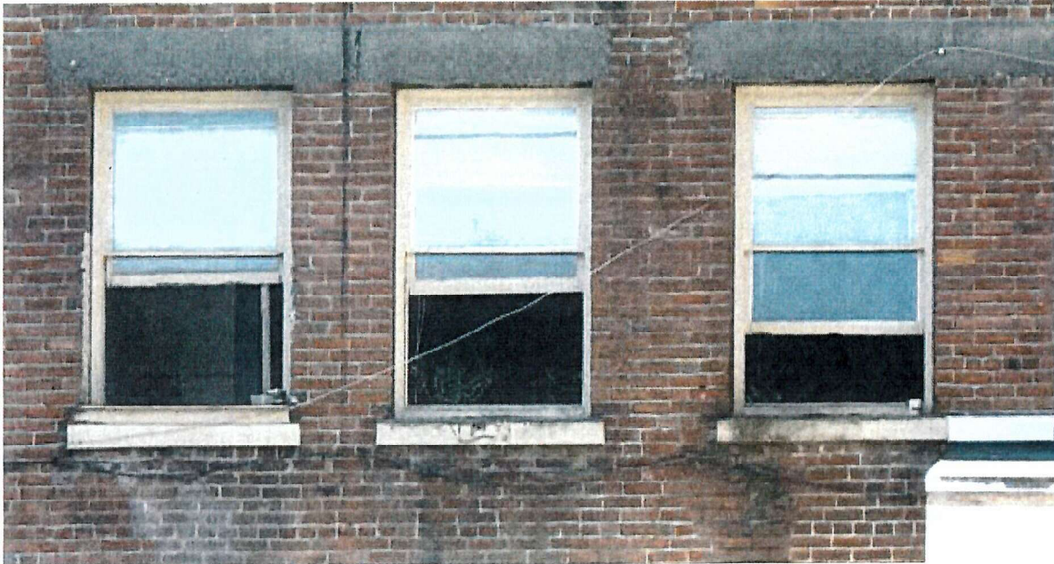
Above: Typical deterioration of masonry on rear of building including staining, cracked bricks, mortar loss, efflorescence and past unsympathetic repairs.
