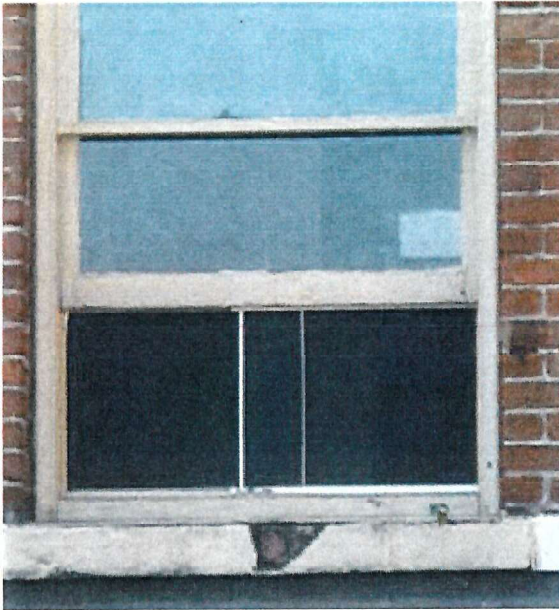
Above: Parge brick sill of rear façade window showing deteriorated parging.
