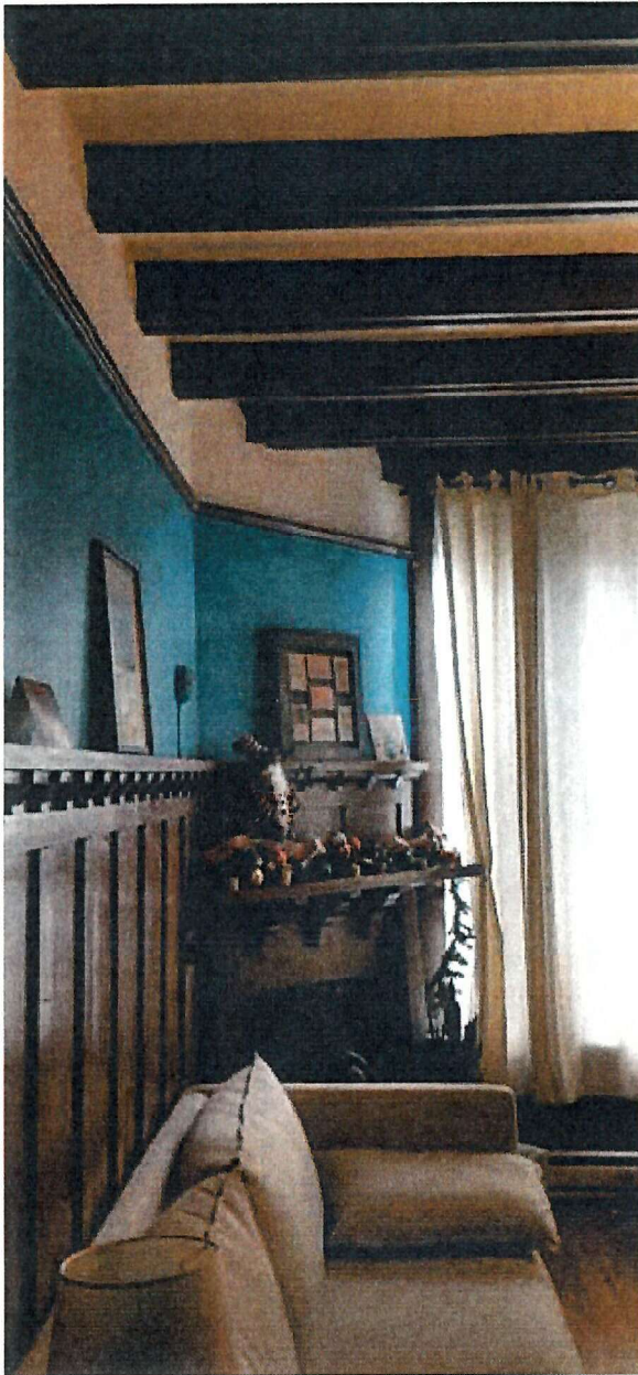
Above Left: Suite interior showing intact wood finishes including floor, trim work, wainscoting, and exposed beams.
