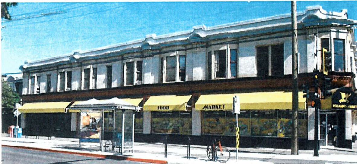
Above and Below: Street façades of Pandora Avenue (above) and Cook Street (below). The building is characterised by its two-storey height, masonry construction, storefront bays, second floor fenestration patterning, storefront and rooftop cornices, parapet, chamfered entry are shown.
