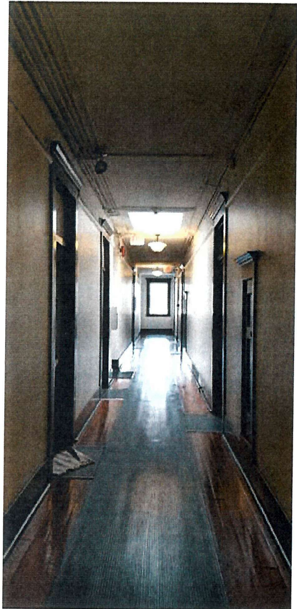
Above: Second floor hallway with intact wood floors, wood doors with transoms, wood trim including casings, baseboards, and picture rail. Rubber runner has been installed.
