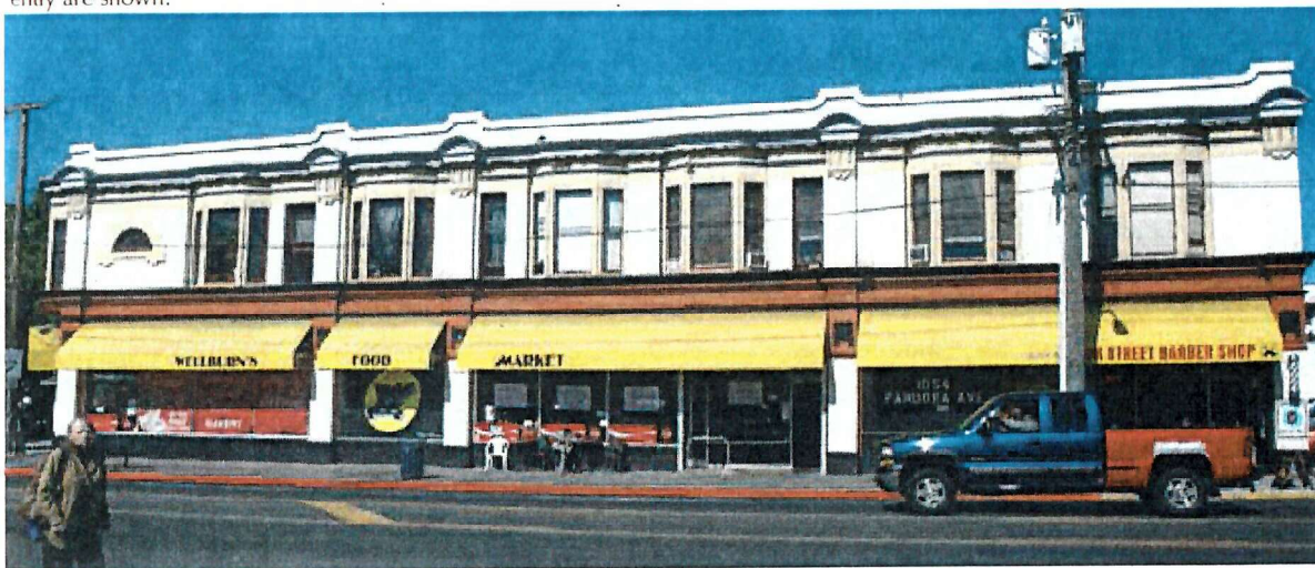
Above and Below: Street façades of Pandora Avenue (above) and Cook Street (below). The building is characterised by its two-storey height, masonry construction, storefront bays, second floor fenestration patterning, storefront and rooftop cornices, parapet, chamfered entry are shown.
