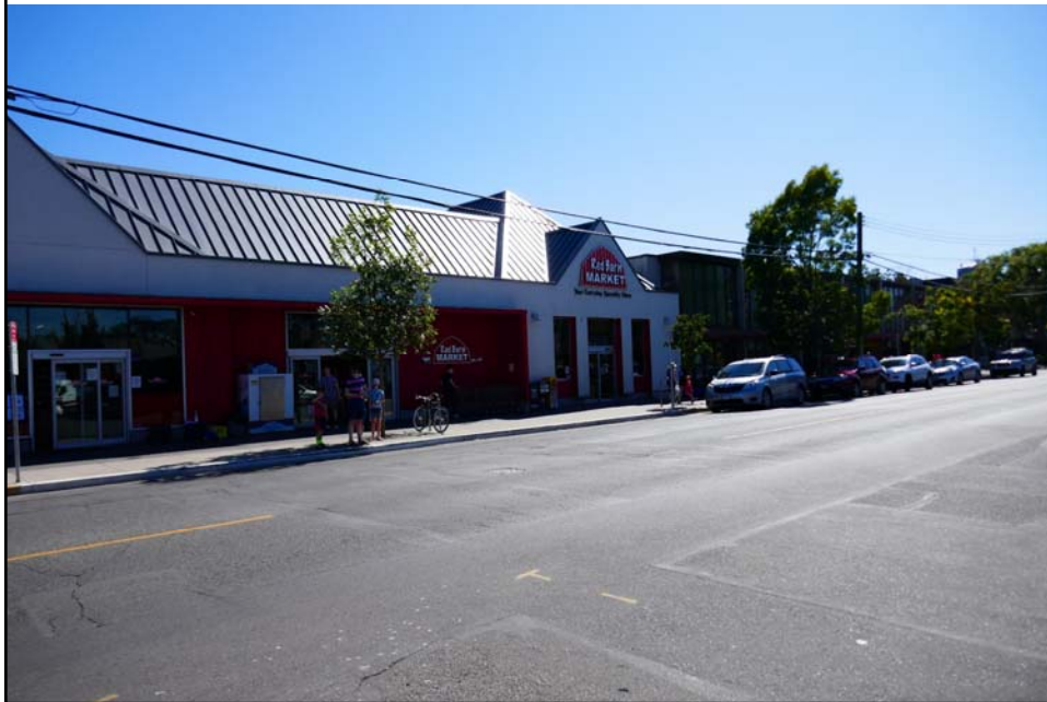
Adjacent Property: 1933 Oak Bay Ave. (south)
