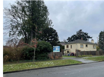
1400 Fairfield Rd. (View from Kipling St.)
