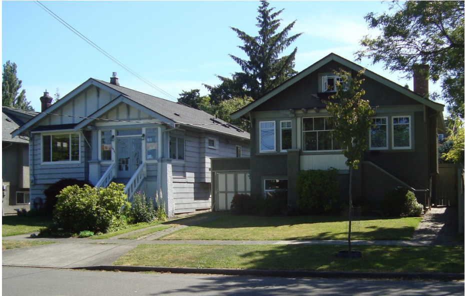
Houses Located Immediately Adjacent to Breia Holdings Ltd. Property on Thurlow Road
