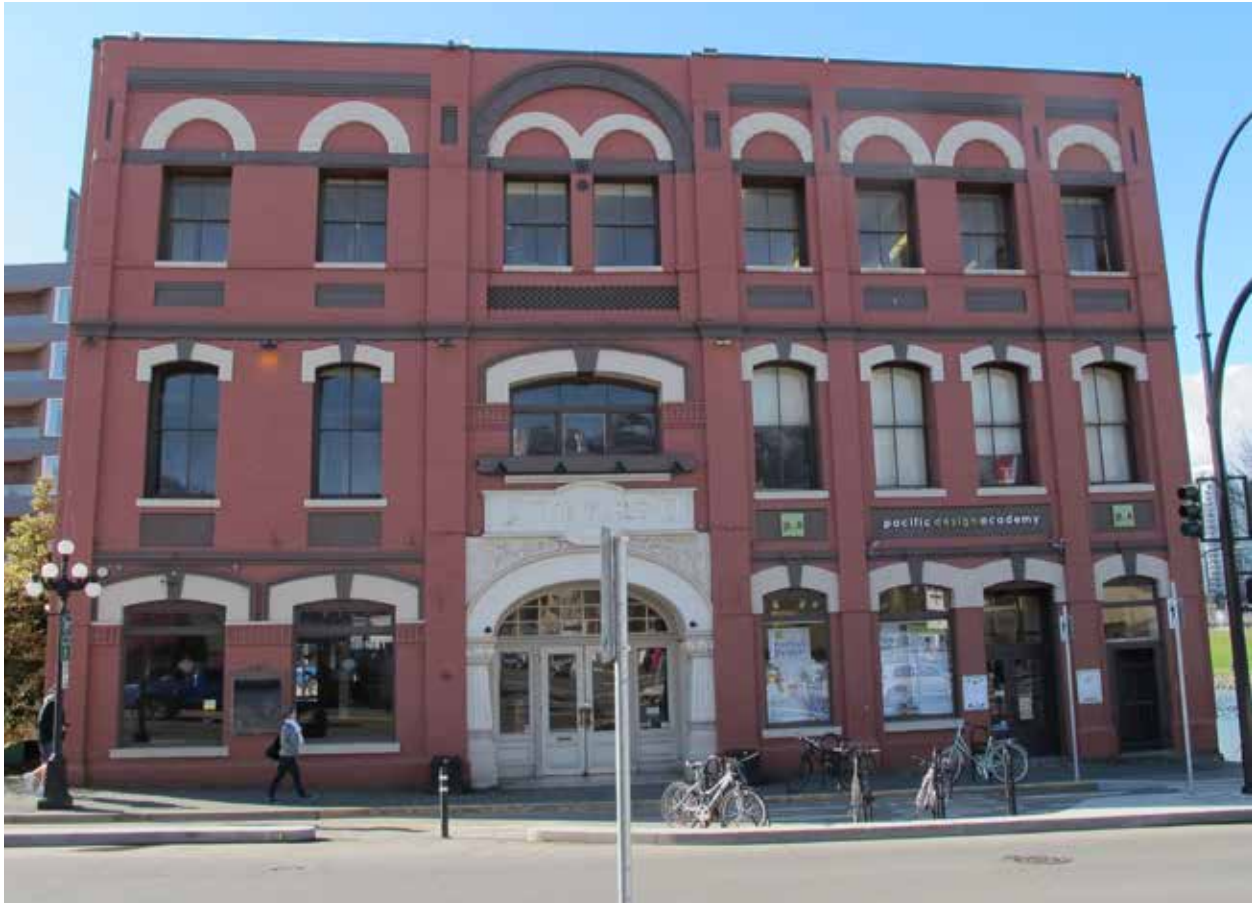
Front elevation of the Yates Block showing multi-wythe brick walls with brick and stone detailing.
