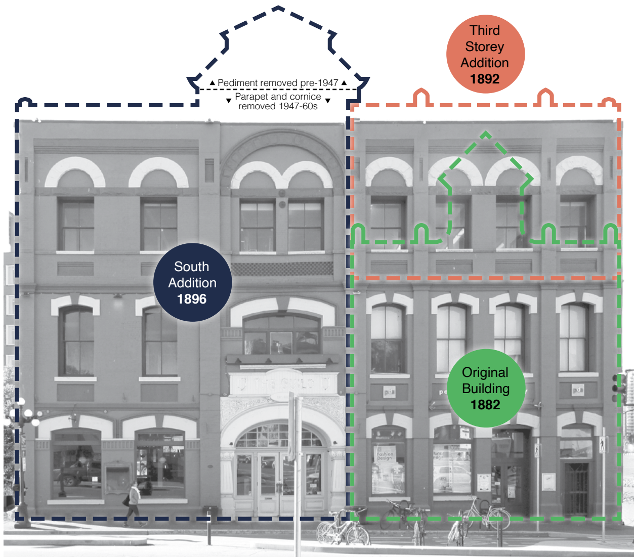
The three primary construction stages of the Yates Block. The pediment and parapet were removed at separate times.
