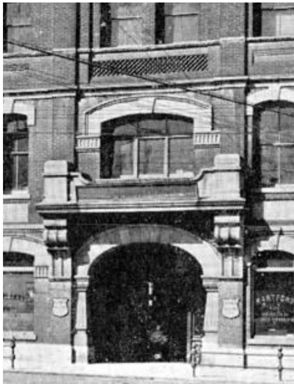
Main entry of the Yates Block following the 1896 addition with balcony supported by large scroll-like brackets.
