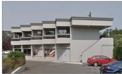
EXISTING VIEW FROM OAK BAY AVE
