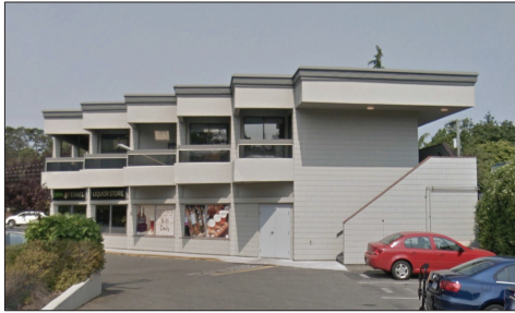
EXISTING VIEW FROM OAK BAY AVE
