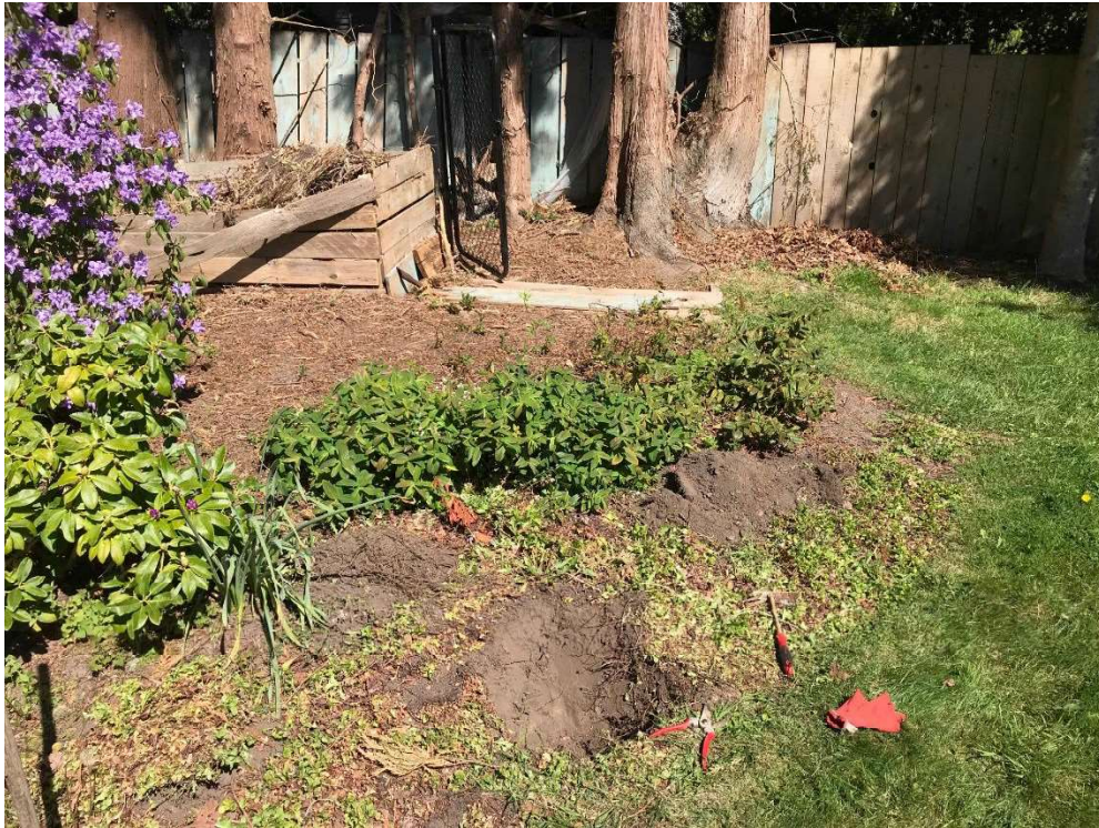
Test hole 4m west from Cedar #208 at approximate location of foundation excavation. One 6cm root was encountered (following picture).
