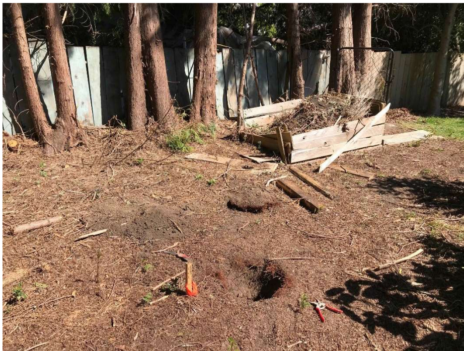
Test hole at patio deck footing location, ~5m from Cedar #207..
