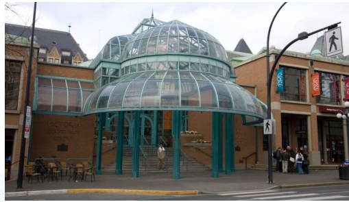
Victoria Conference Centre– 750 Douglas St.
