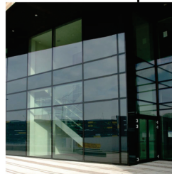
LEVEL 1 LOBBY -SSG W/BLACK SEALANT
