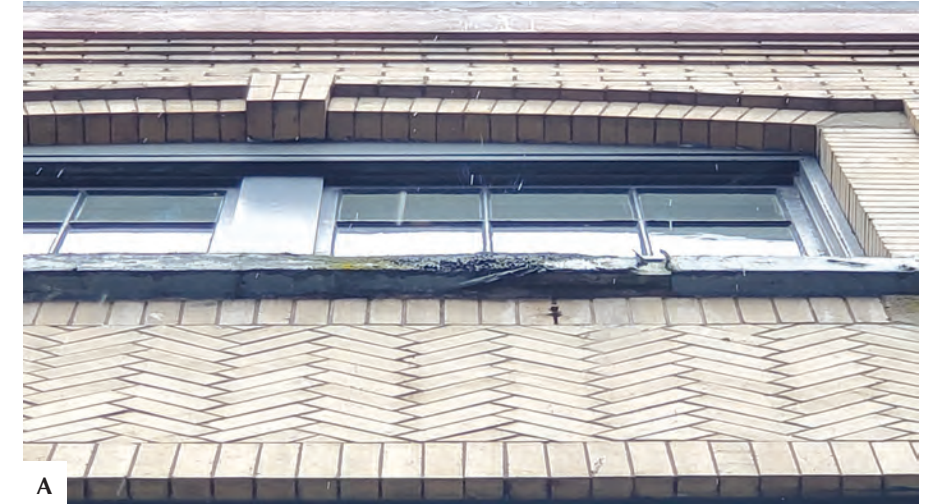
Figure 29: Detail photo showing typical deterioration of window sill. Note discolouration and biological growth, and paint failure.
