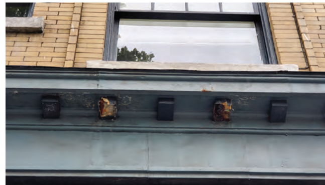
Figure 24: Detail photo showing existing typical deteriorated condition of storefront metal cornice.
