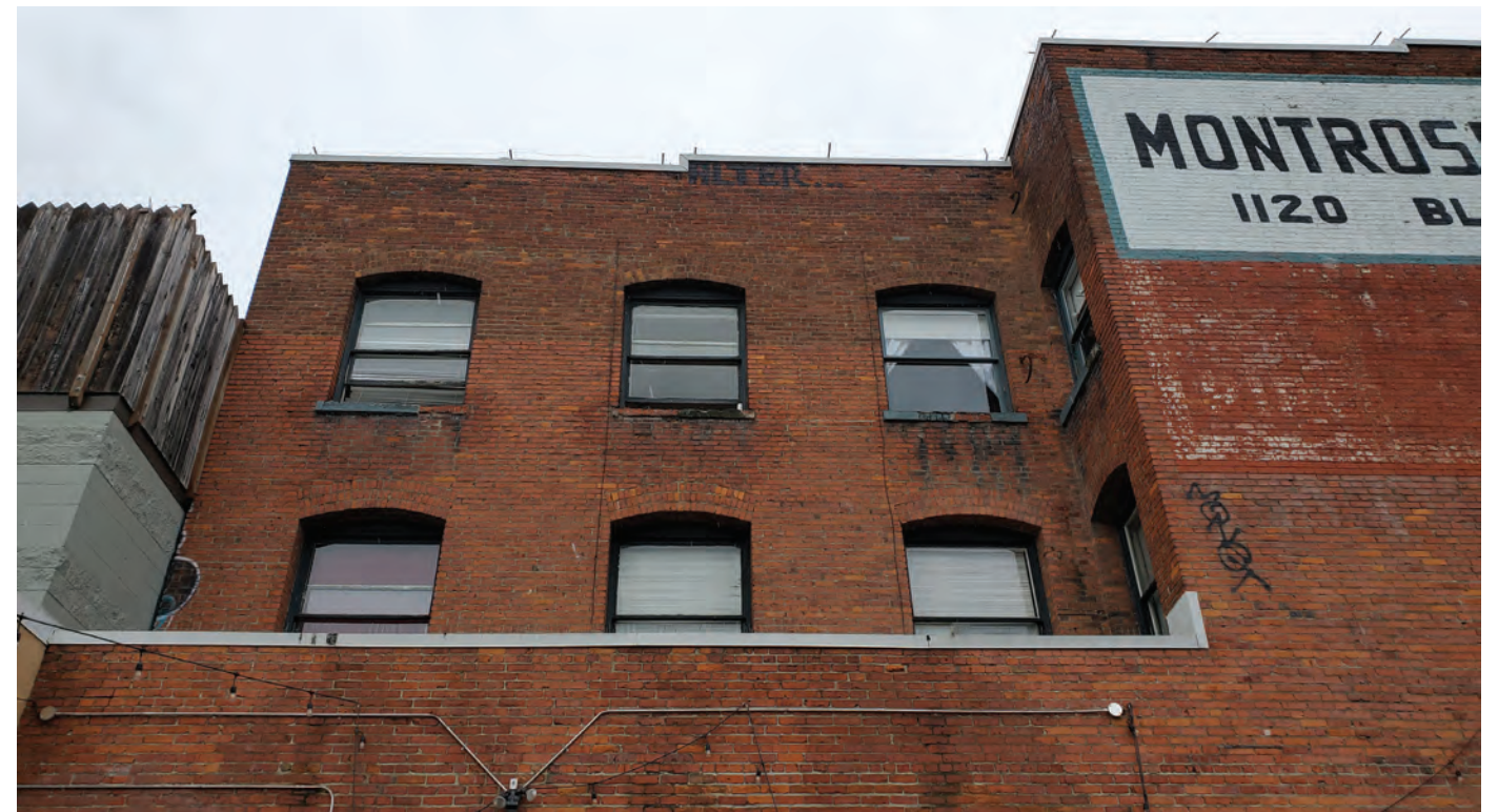
Figure 21: Detail photo showing arched window openings with double-hung wood window sashes at south elevation. Note deteriorated parging of wood window sills, exposing brick masonry units in rowlock coursing underneath.
