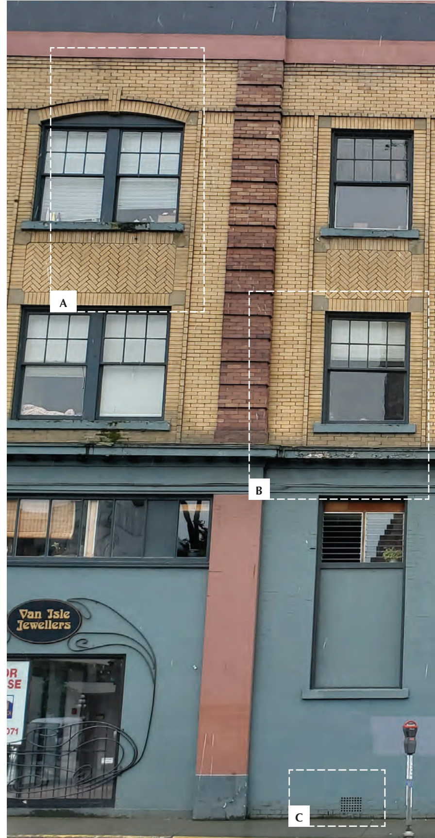
Figure 28: Detail photo showing partial North Elevation (along View Street) showing typical deterioration of exterior character-defining elements caused by water ingress and saturation.
