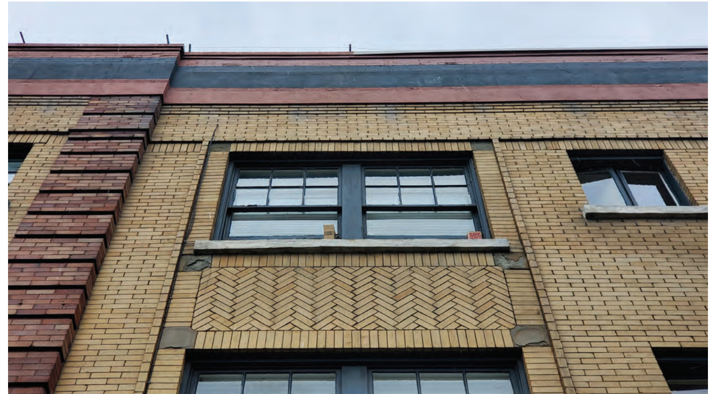
Figure 20: Detail photo showing typical paired wood window assembly with double-hung sashes. Note typical deterioration of brick masonry units below missing parapet cornice.
