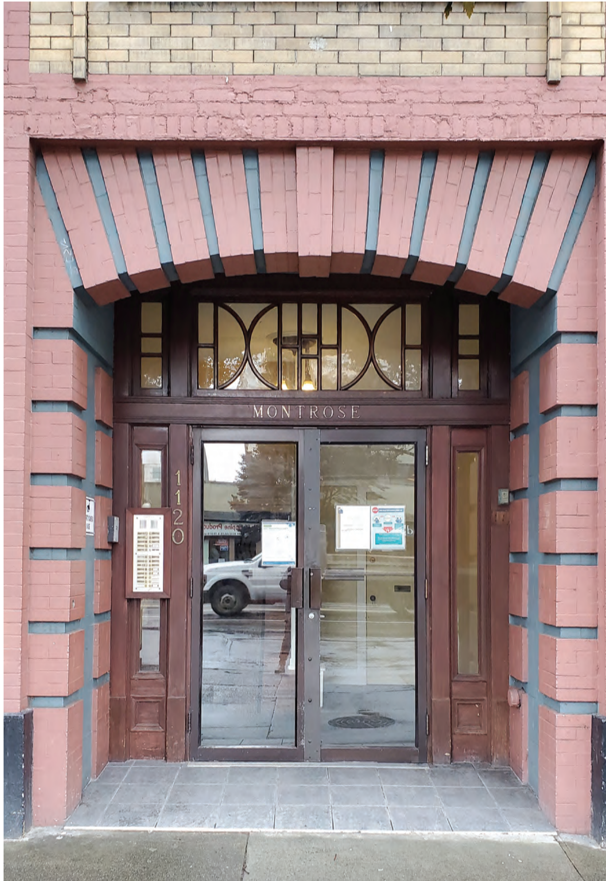
Figure 22: Detail photo showing recessed primary entrance portico at central bay of front facade along Blanshard street. Note existing replacement door sashes (paired narrow-stile metal doors with glass inset) that are not historically appropriate.
