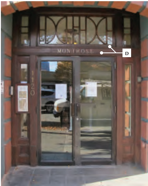
Figure 13: (Left) Primary Entrance Wood Door Assembly
