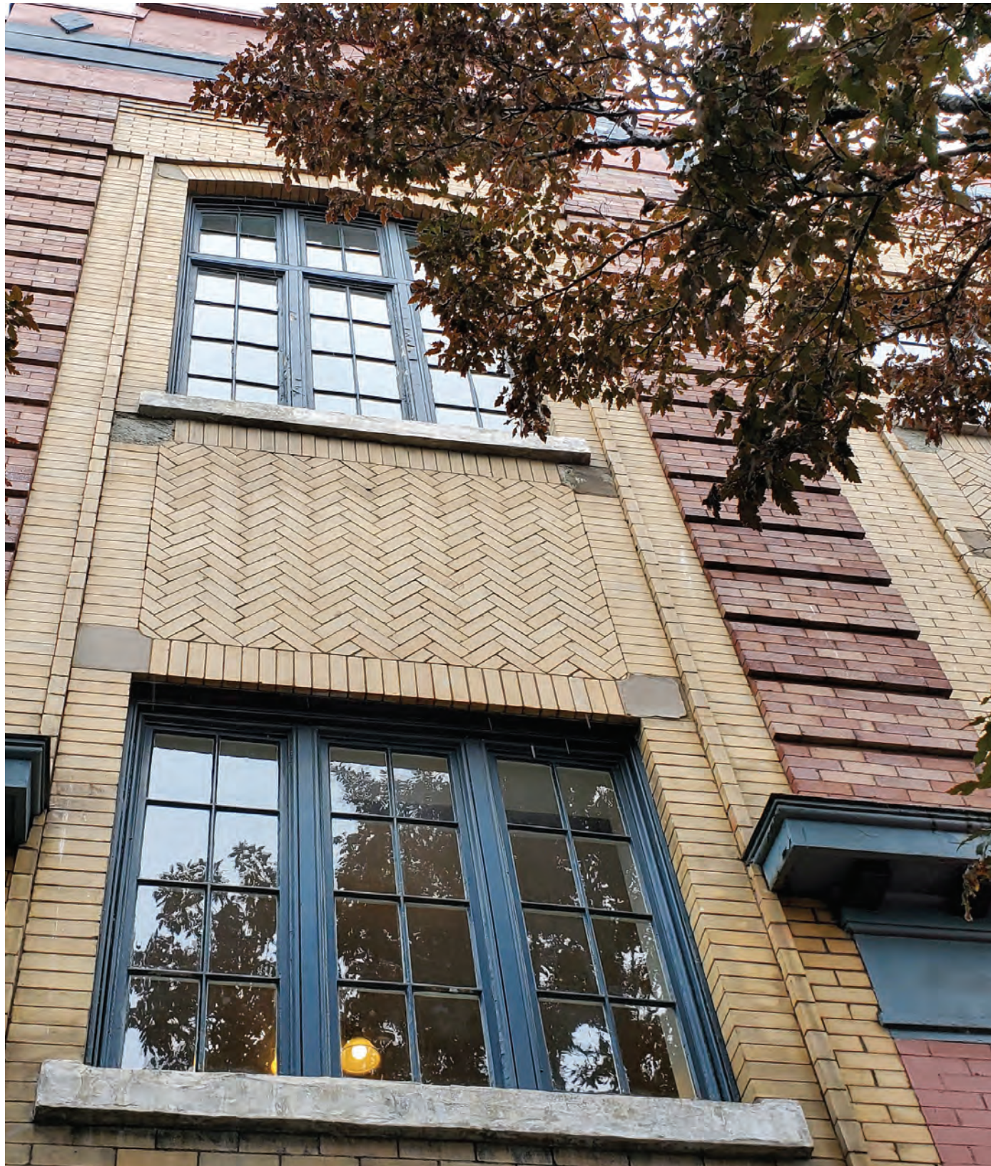
Figure 19: Detail photo showing central bay above entrance alcove. Note typical deterioration of window sills, sandstone insets, and wood window frames.
