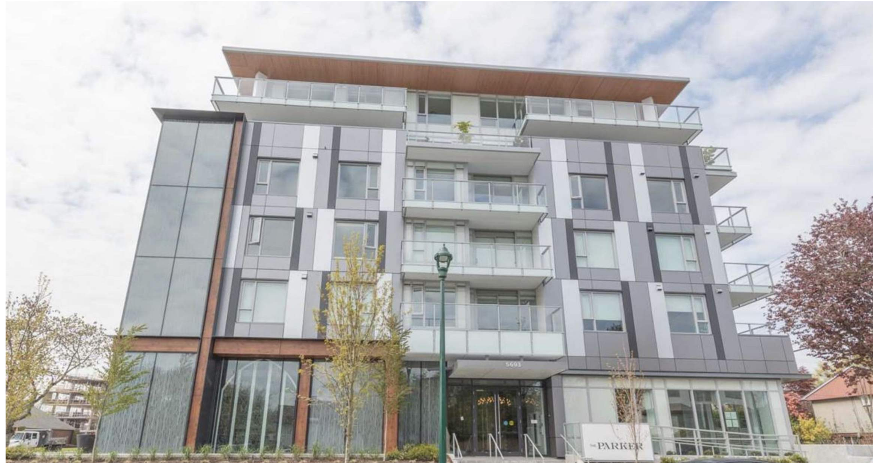
Aluminum and phenolic wood panels precedent
