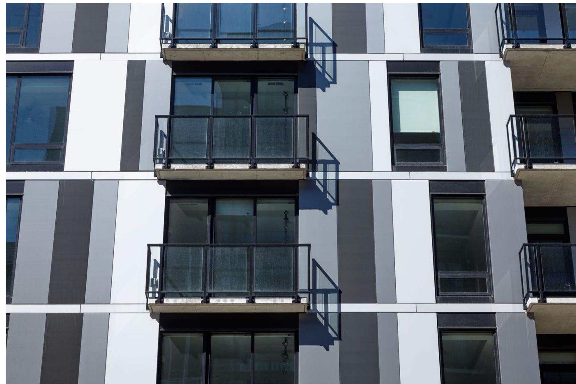
Aluminum composite panel precedent Product proposed: Stac Bond or similar Colors: Signal white, Light grey, Silver metallic, Titanium metallic, Carbon Finishes: Matte - Acabado and Metallic
