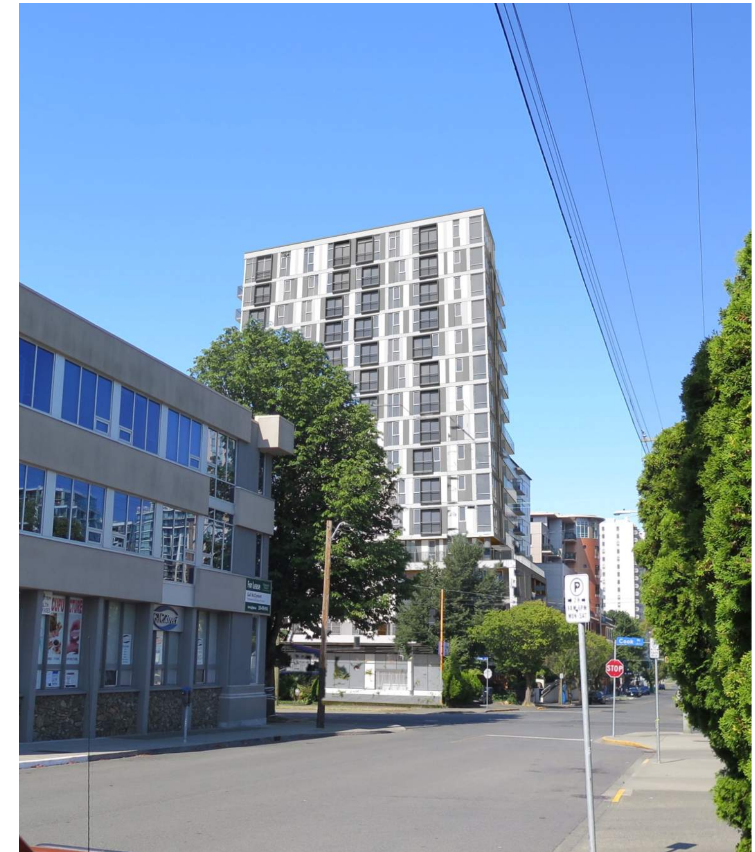
D View Street Looking West
