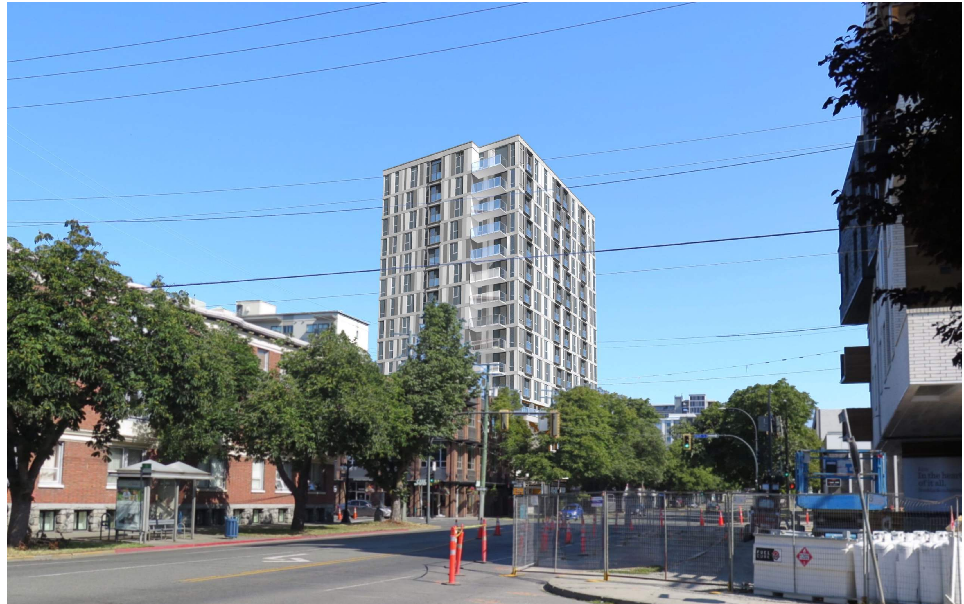
A Cook Street Looking North
