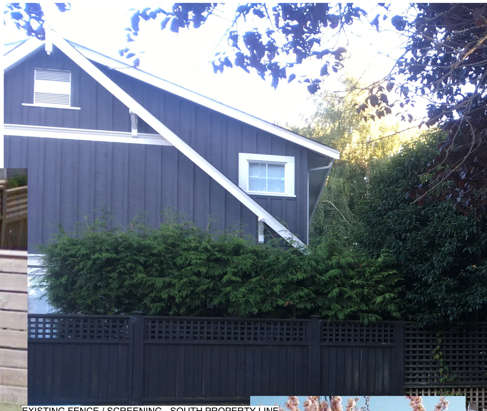
EXISTING FENCE / SCREENING - SOUTH PROPERTY LINE PANEL 5 FT HEIGHT T&G VERTICAL BOARDS W/ LATTICE ABOVE - STAINED
