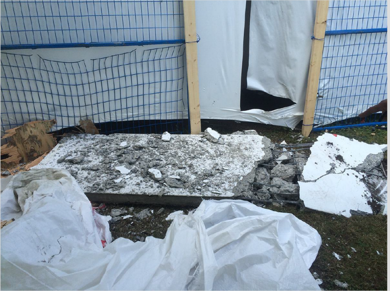
Concrete slab landed by entrance to enclosure
