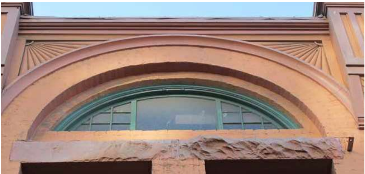
Top: Photo showing typical existing condition of original double-hung wood window assembly with transom light.
