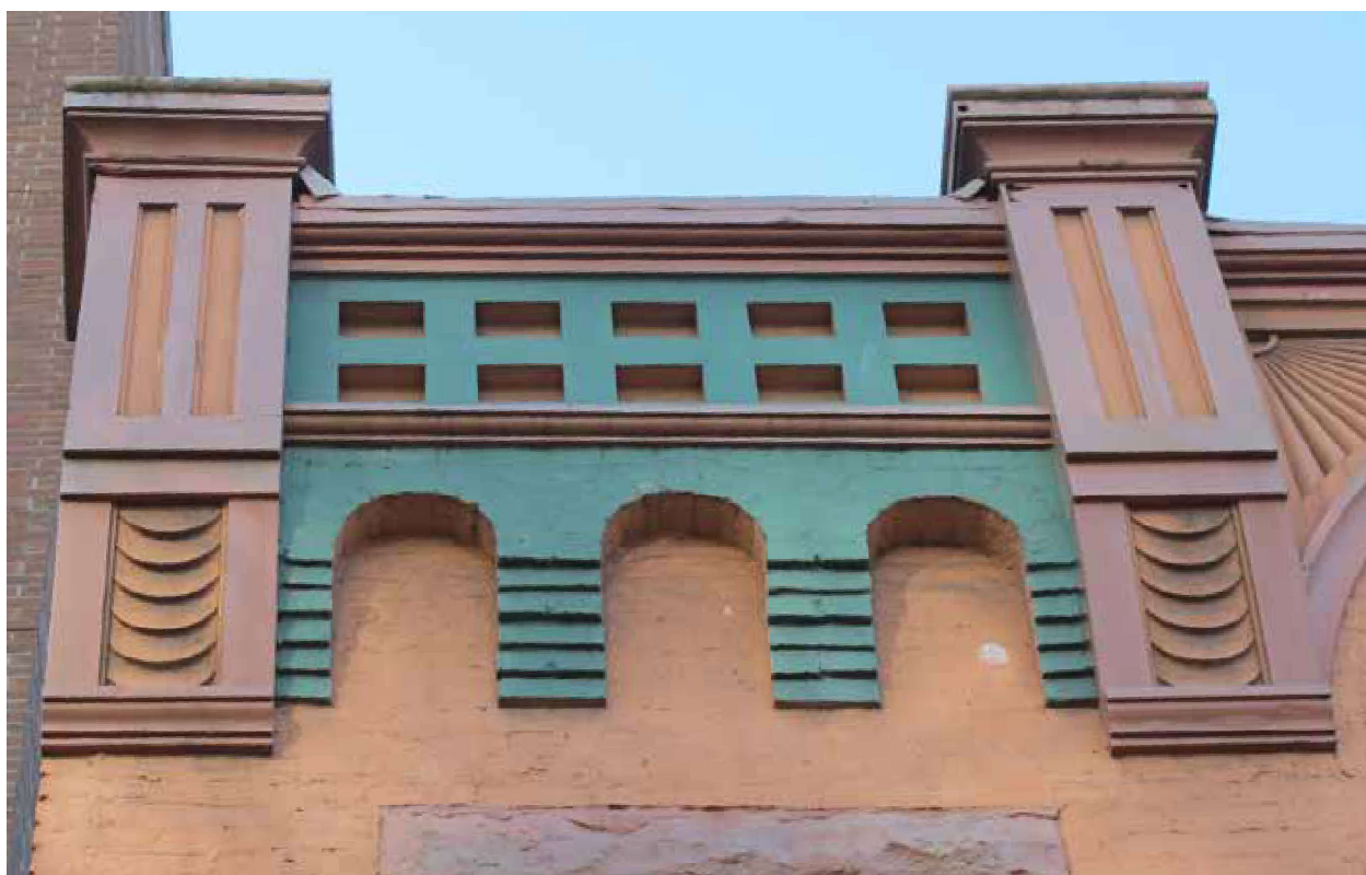
Existing condition of rehabilitated architectural metalwork that resembles original based on archival photos.
