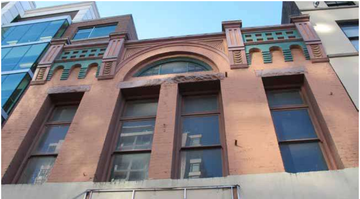
Detail photo showing existing condition of the masonry elements and architectural metalwork above storefront level of the historic front facade. Note existing parged concrete cladding at window sill to be removed.
