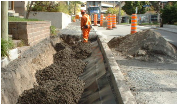
Structural soil installation
