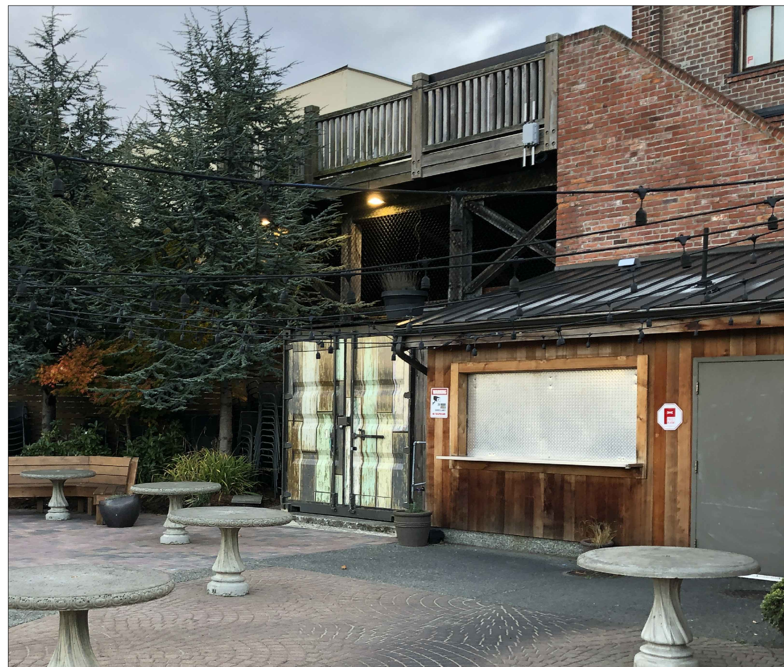
04 A405 EXISTING SITE PHOTO NTS
