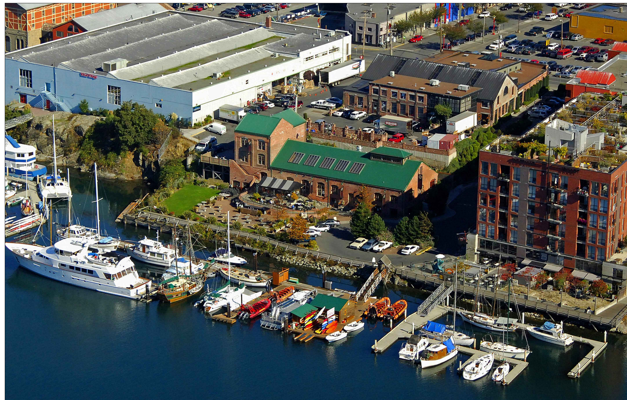
01 A405 EXISTING SITE PHOTO NTS
