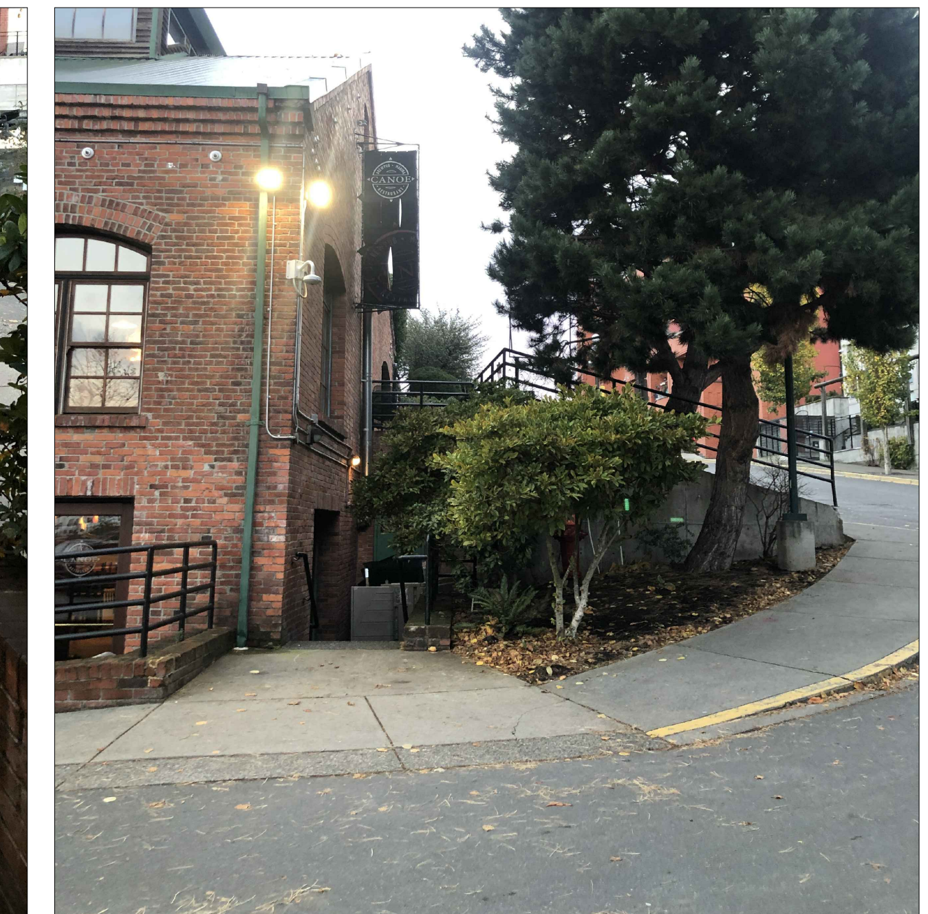
07 A405 EXISTING SITE PHOTO NTS
