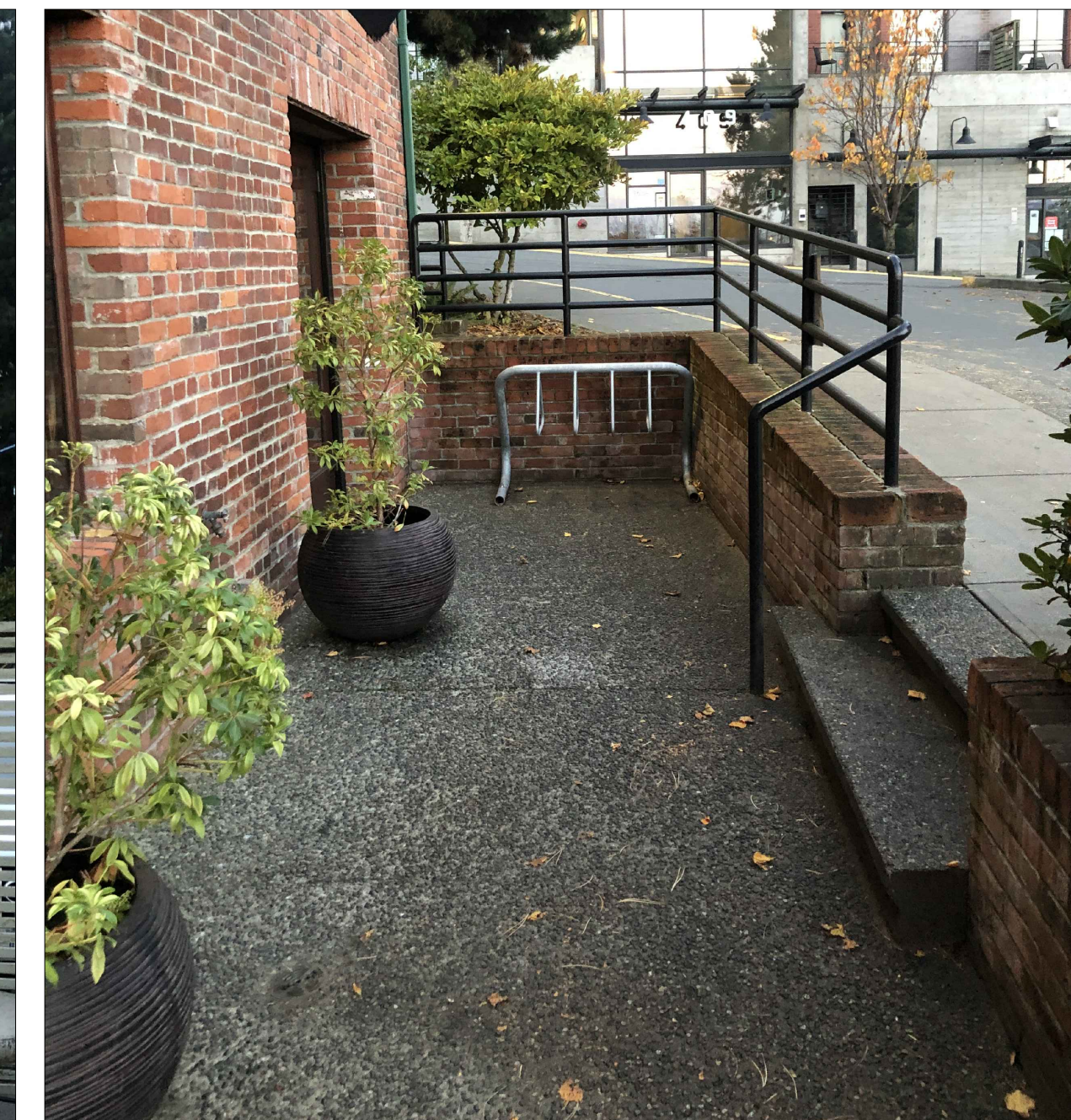
06 A405 EXISTING SITE PHOTO NTS
