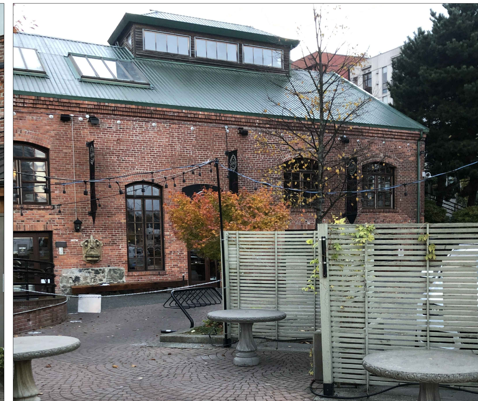
05 A405 EXISTING SITE PHOTO NTS
