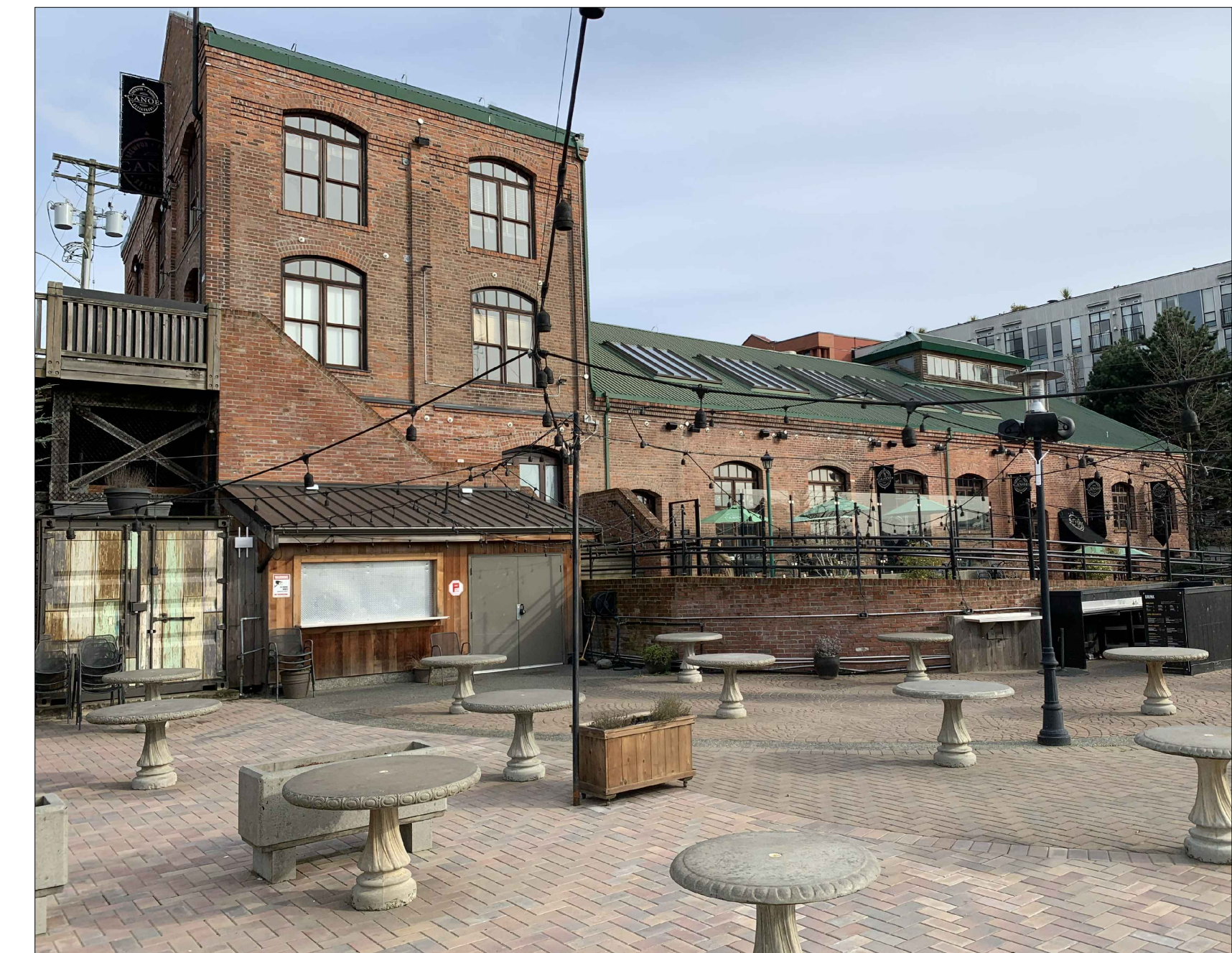
03 A405 EXISTING SITE PHOTO NTS
