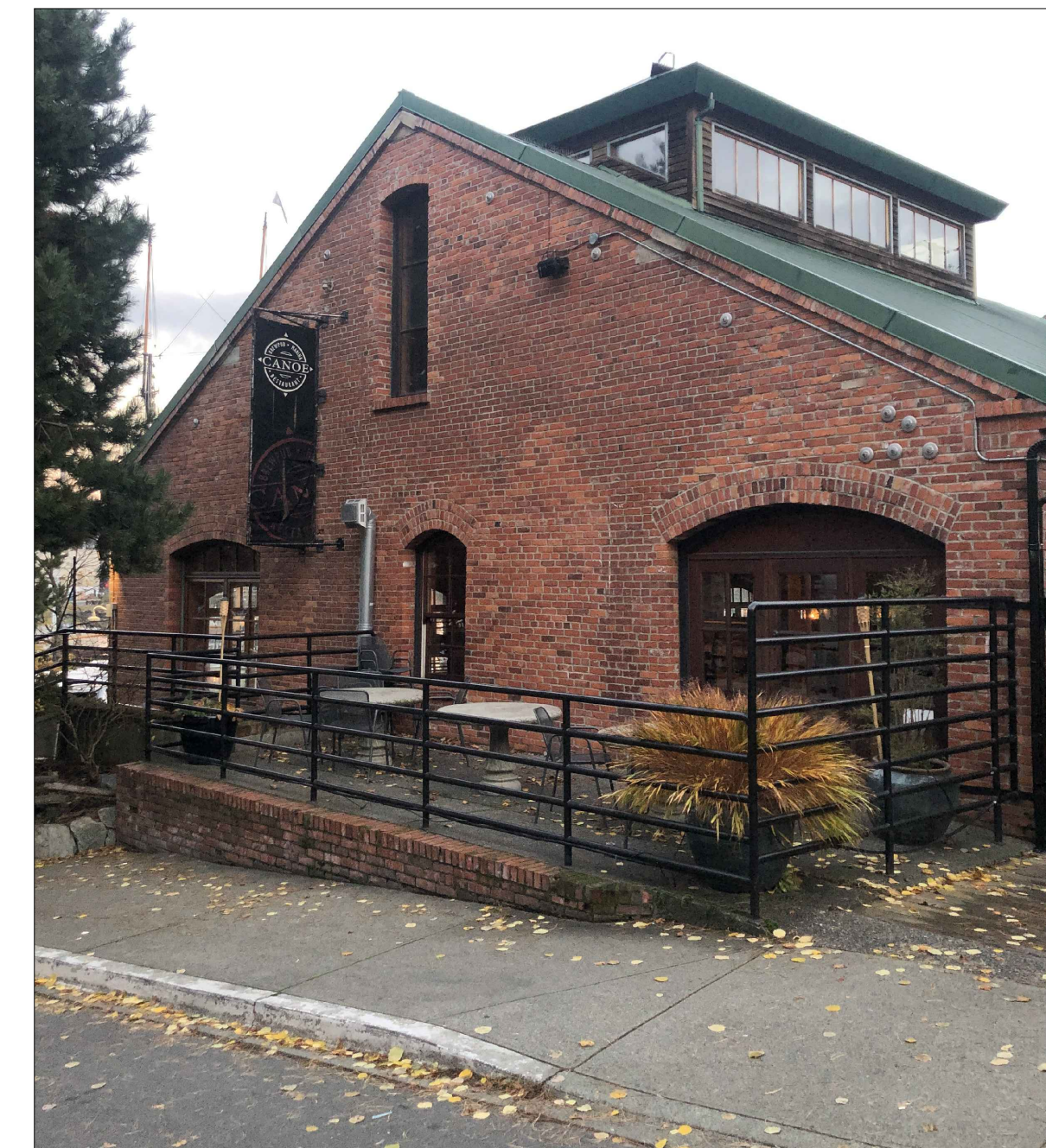
09 A405 EXISTING SITE PHOTO NTS
