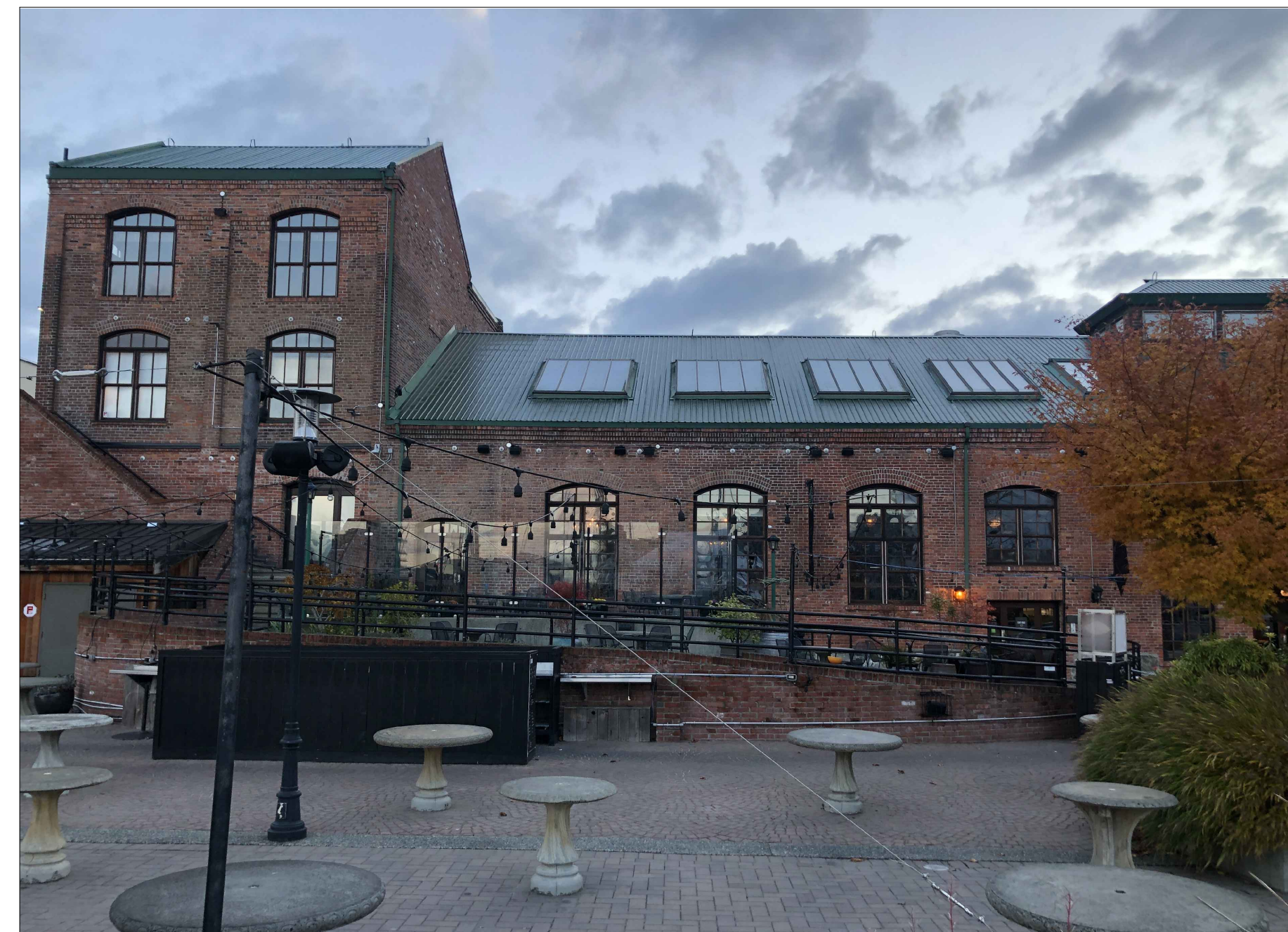
02 A405 EXISTING SITE PHOTO NTS
