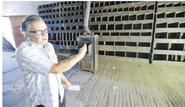
Reliance Properties CEO Jon Stovell says the plan is to keep the historic warehouses' outer walls and an inner wall, made of a mix of brick and stone rubble, while replacing the rotted floors and ceilings. The walls would be reinforced and seismically upgraded to support added stores. ADRIAN LAM, TIMES COLONIST
