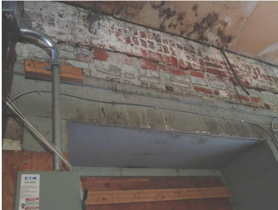
Segmental arch above altered front opening
