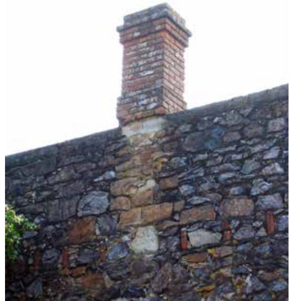
Parapet And Chimney at Rear of Building - No Cap Flashing Noted
