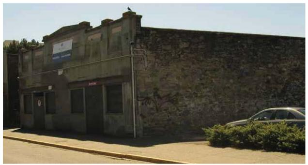
Current front elevation with late applied stucco of the Fraser Warehouse.
