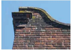
Parapet at rear of Building - no cap flashing noted
