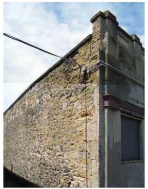
Current side and front elevations showing the stone construction with quioning on the corner Fraser Warehouse
