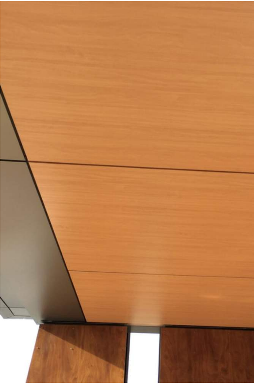
Phenolic panel precedent Product proposed: Gentas or similar Reference: 4600 Velur Texture: Wood Finish: Smooth
